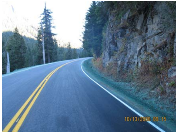
A road in Mt Rainier National Park. WFLHD Construction Archives.
