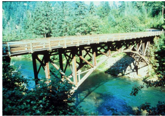
A recent view of Mott Bridge on the Umpqua River. WFLHD Archives.
