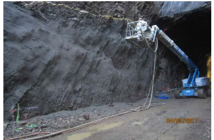
DURING SHOTCRETE APPLICATION
