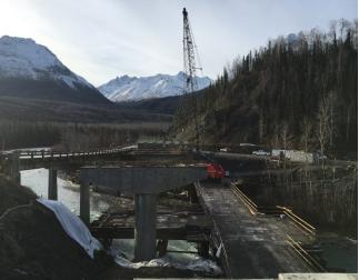
It took five separate deck pours to complete the bridge deck. The cast-in-place concrete deck serves to stabilize the structure.
