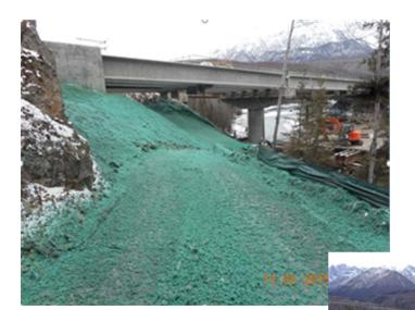
Hydroseed was blown around the surrounding area to ensure ground stabilization throughout the extreme winter weather conditions while the project construction was shut down.
