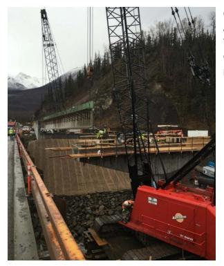
Girders for the new bridge were trucked in from Anchorage, after being barged up from Seattle, Washington. The size of the girders was such that two cranes were needed to set them in place, each crane picking up one end of the girder.
