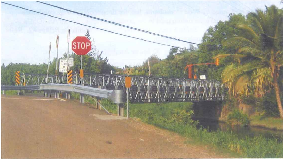
Photo 11 : Current Bridge #2 - ACROW Panel Bridge (no Queen Post Truss)
