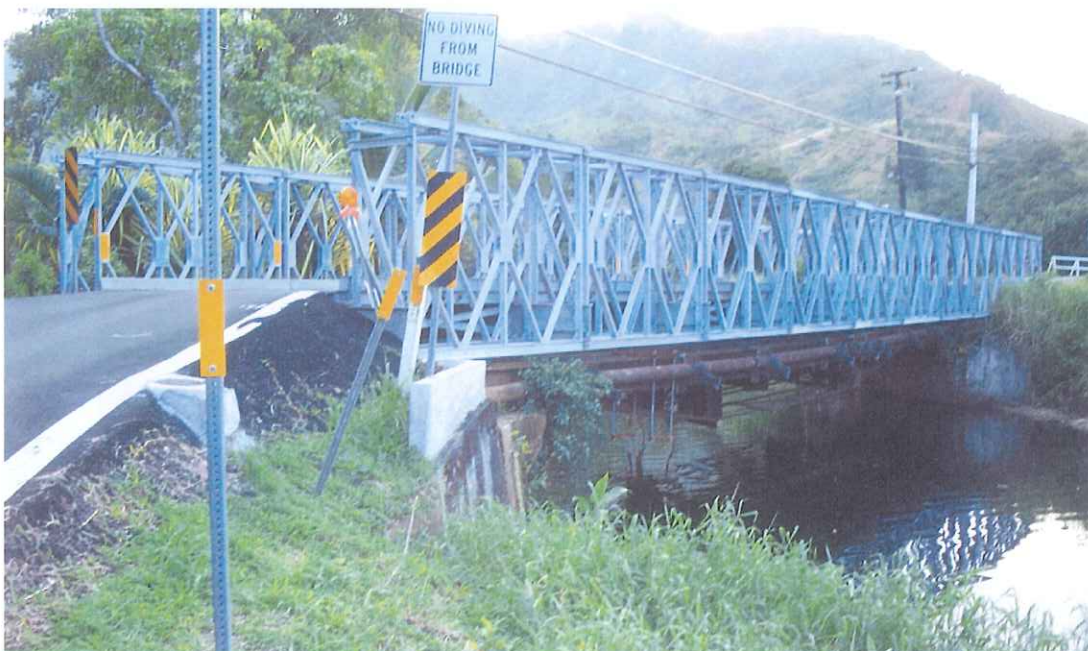
Photo 10 : Current Bridge #2 - ACROW Panel Bridge over Queen Post Truss
