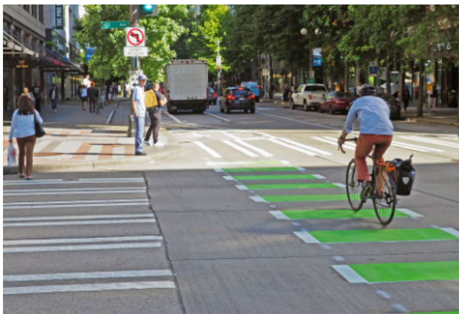
Figure 4. Example of roadway characteristics factor. The cross-sectional elements of this road include sidewalks, parking, and bicycle lane.
