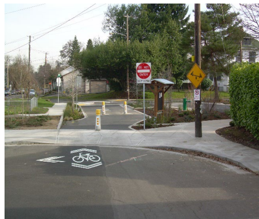
A street was closed and a small park expanded, with bike access preserved, for a bikeway project. (Source: PBOT)
