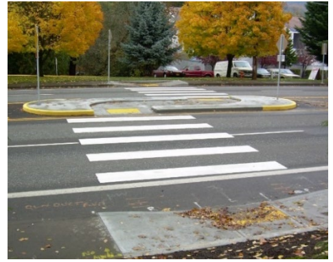
A refuge island with a Z-crossing that directs the pedestrian to focus on oncoming traffic before they enter the roadway from the island. (Source: PBOT)
