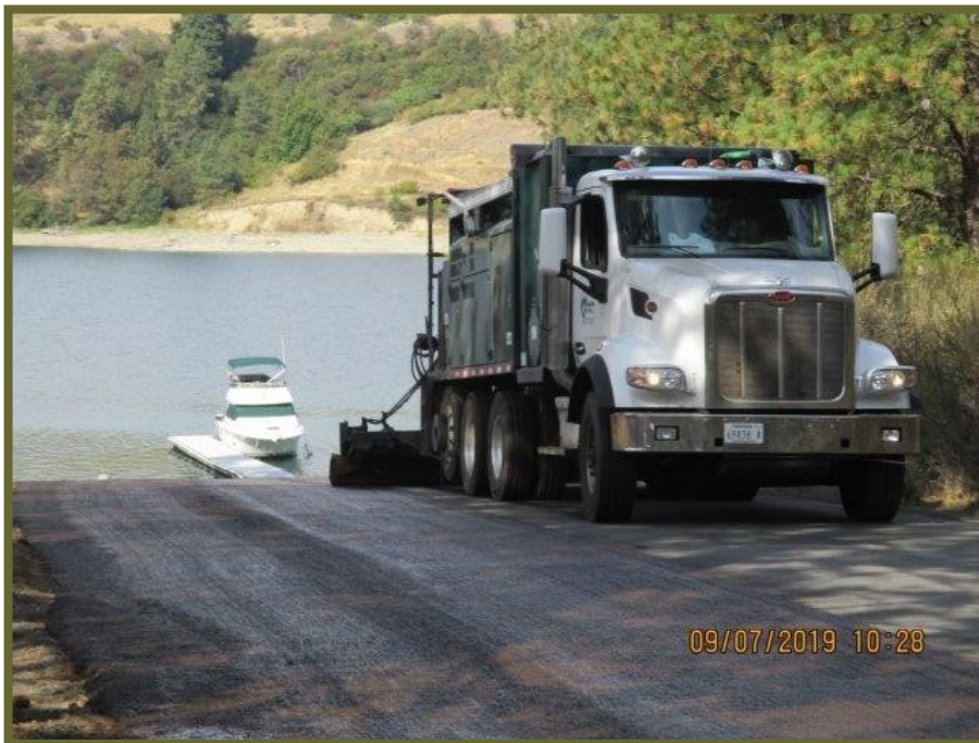
Micro Surfacing Ft Spokane Boat Launch
