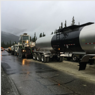
Beginning the FDR control strip.
