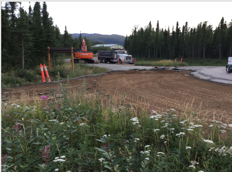
Removing the asphalt at the round-about.
