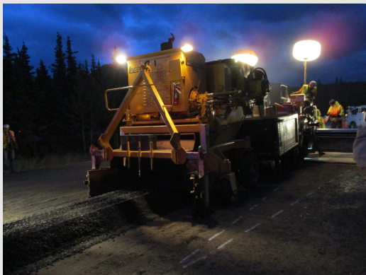
Front view of paving operations.
