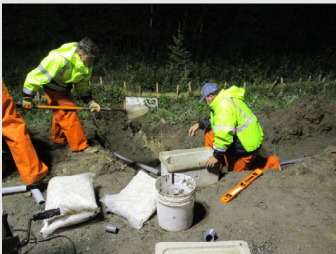
Installing pull boxes for the traffic counter system.
