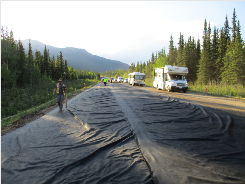
Placing fabric on the subex.
