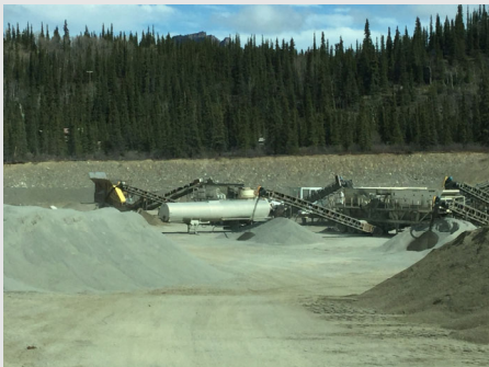
Pruhs Construction producing material at the MP 230 pit.
