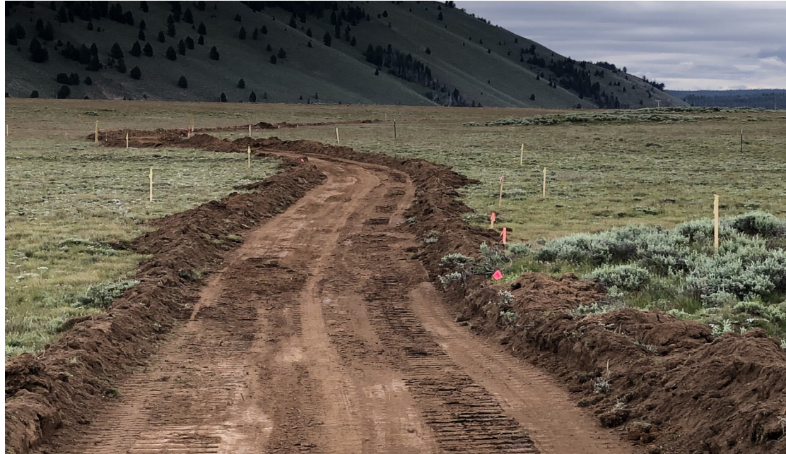
Preparing Subgrade for trail.
