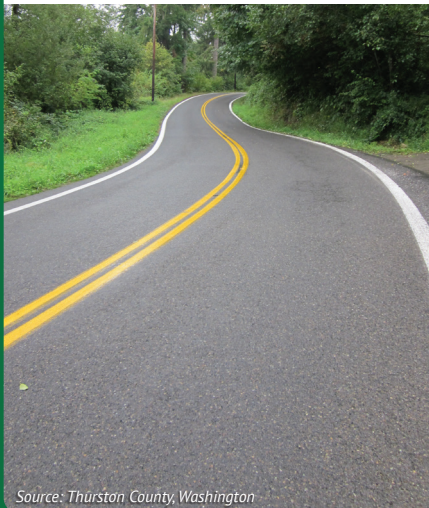
Source: Thurston County, Washington
