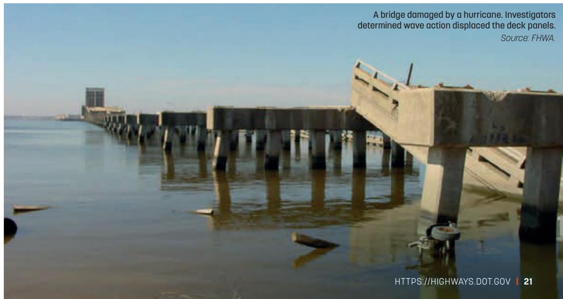
A bridge damaged by a hurricane. Investigators determined wave action displaced the deck panels.
