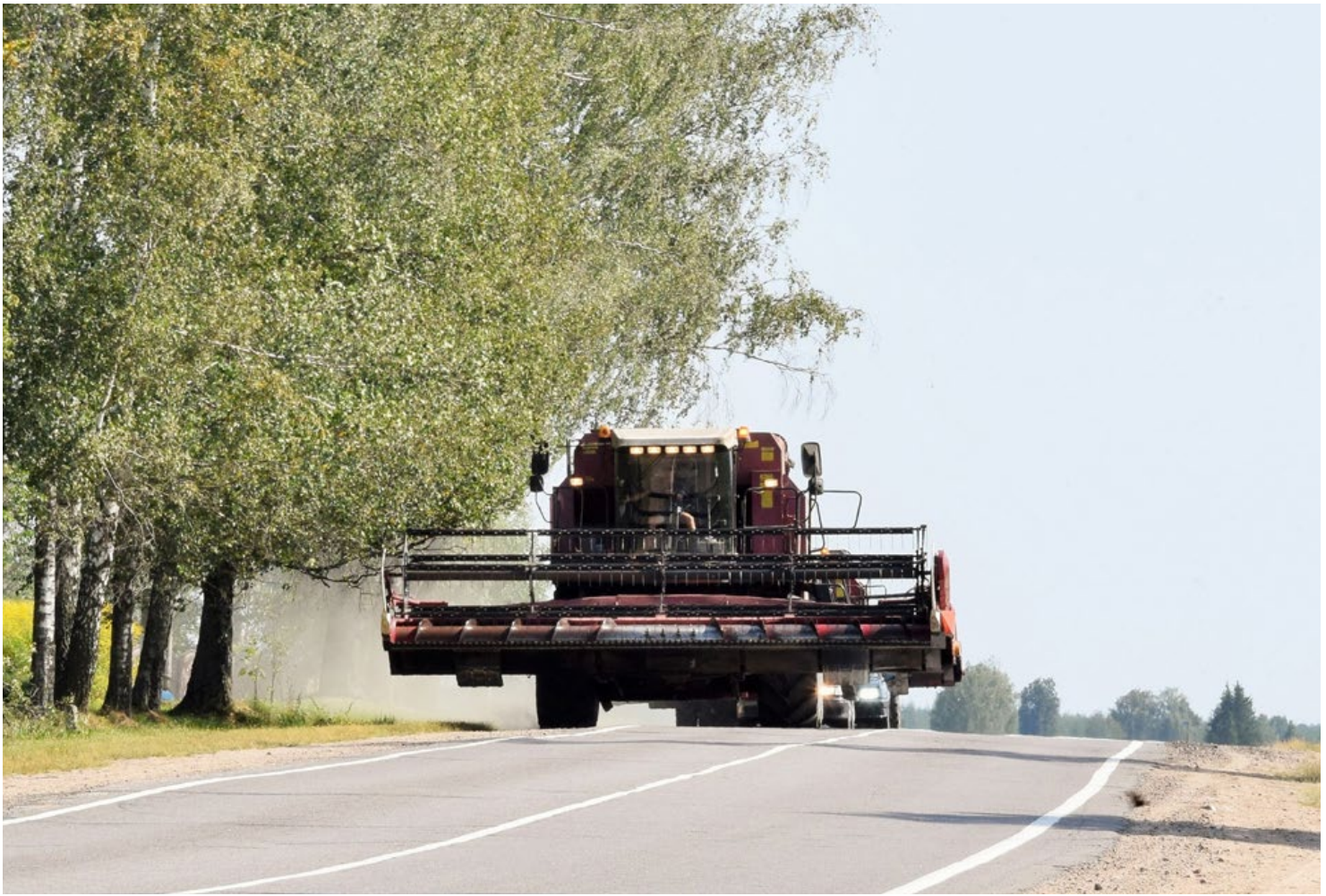
Lack of pull-off areas on narrow rural roads result in an increased potential for road departure incidents or collisions.
