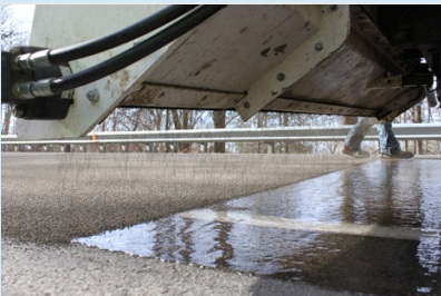
Automated application of HFST. Source: FHWA
