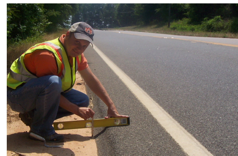
Example of the SafetyEdge SM after backfill material settles or erodes. Source: FHWA
