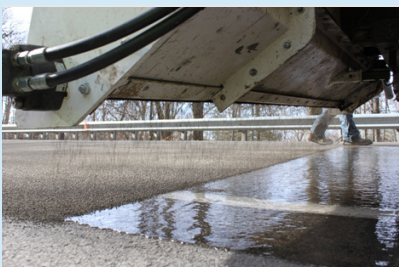
Automated application of HFST. Source: FHWA
