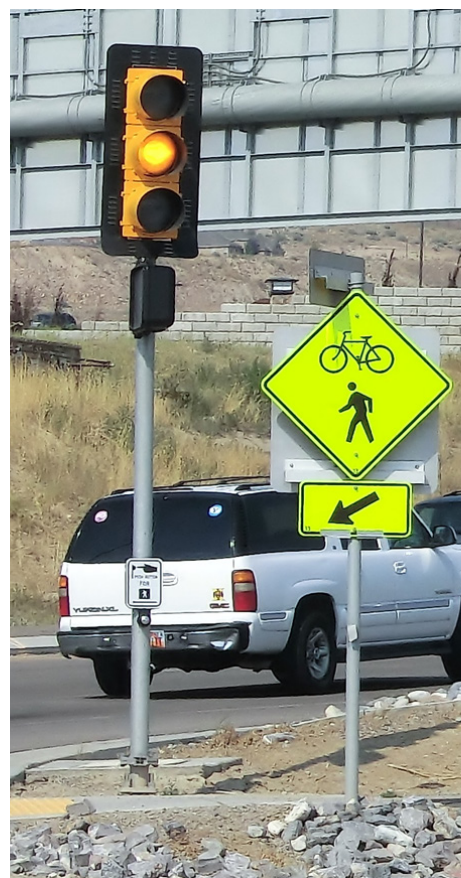
Appropriately timed yellow change intervals can reduce red-light running and improve overall intersection safety. Source: FHWA
