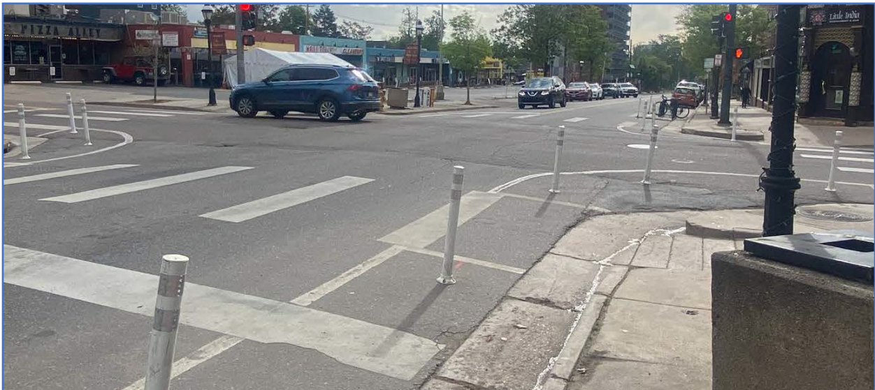
Figure 3: A rapid response countermeasure to install daylighting with flexible delineator posts in commercial area with heavy pedestrian volumes with the goal “to slow vehicles and shorten the crossing distance”
