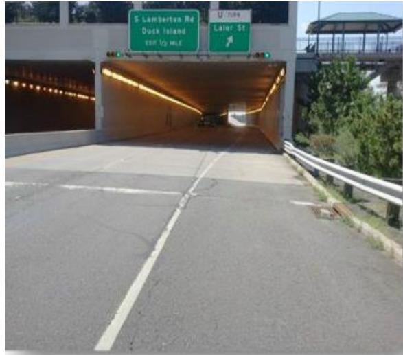
A view of the approach zone to a tunnel.
