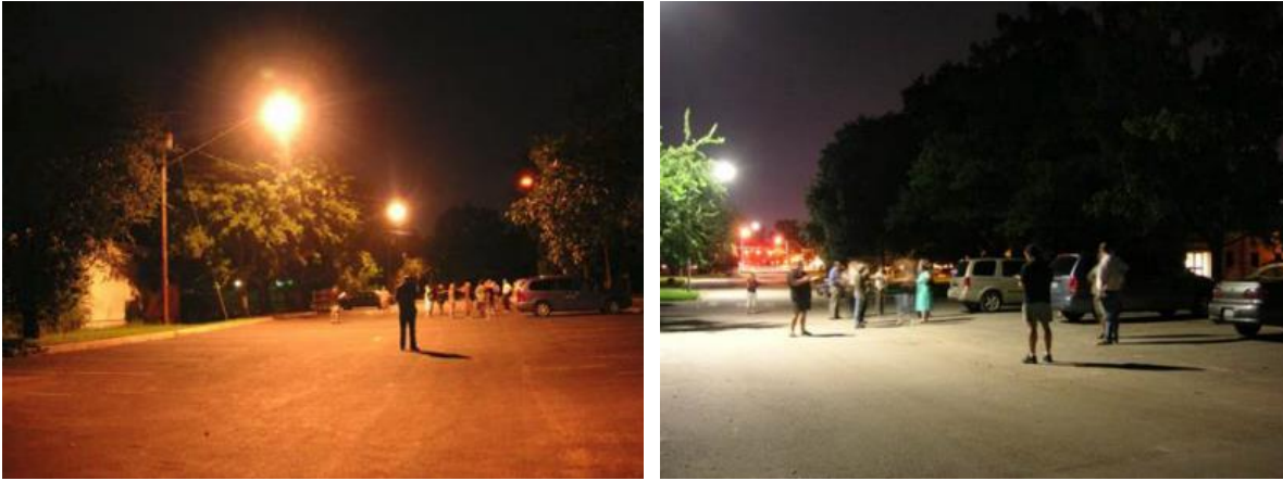
An HPS installation (left); a white light source installation (right).
