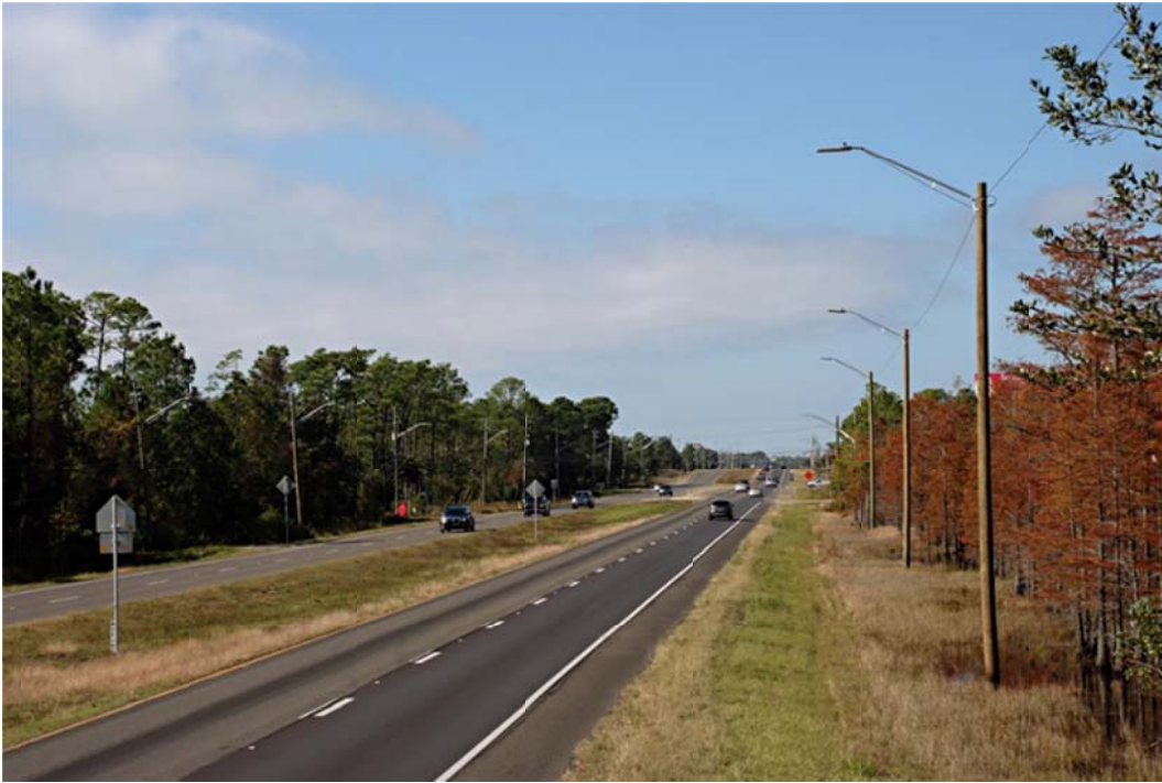
Light poles placed at the end of the clear zone along a highway.
