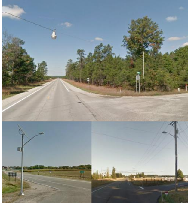
Examples of beacon lighting at rural intersections.
