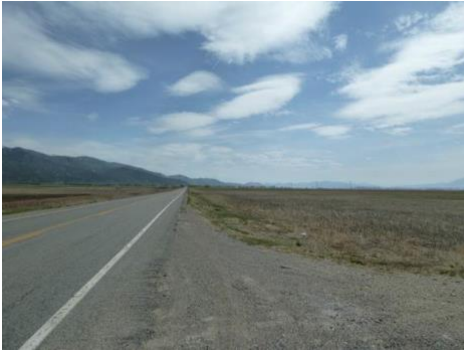
A clear zone on the side of a rural highway.
