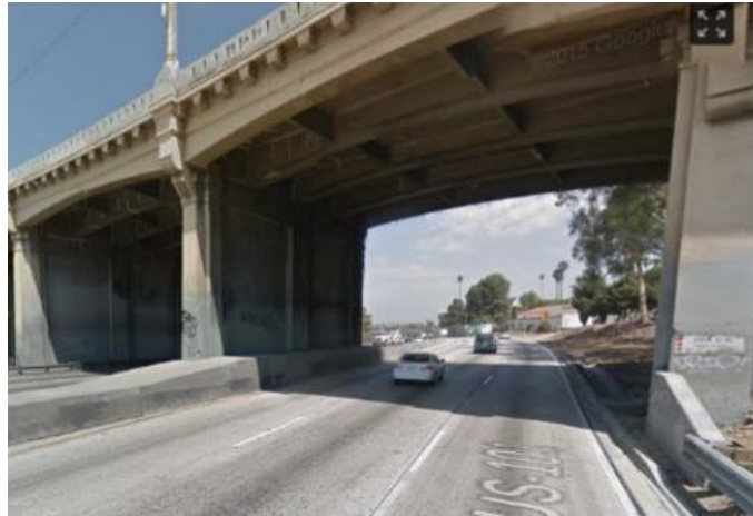
A typical highway underpass that might require lighting.
