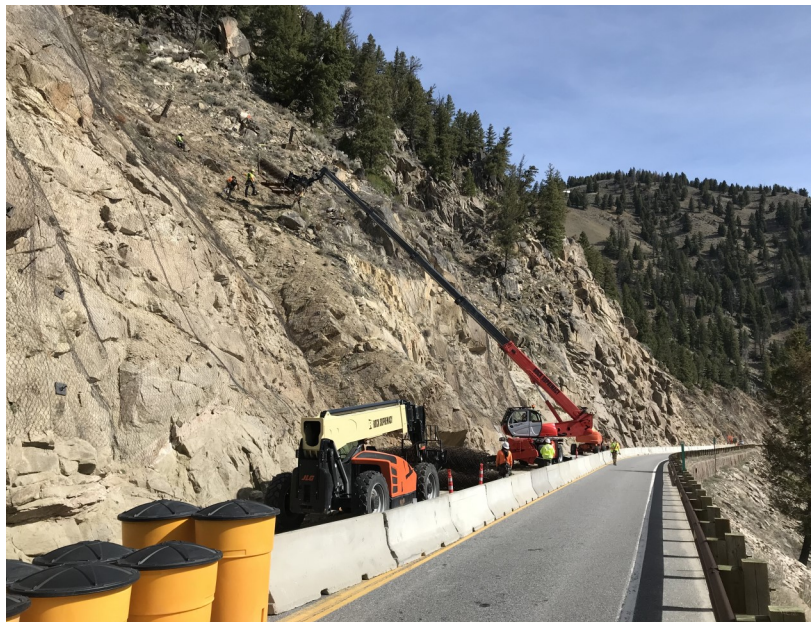
Unrolling Attenuator Mesh in Section 5
