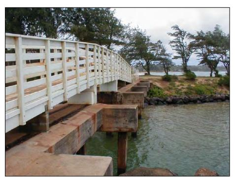
Figure 16. Close-up of Waika'ea Bridge, pedestrian bridge built over railroad bridge, view to northeast (CSH 2002)
