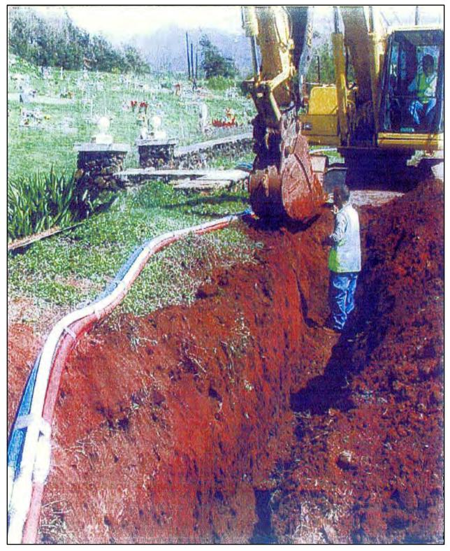
Figure 24. Excavation of trench for fiber-optic cable running along west shoulder of Kūhiō Highway near the current project APE (Dega and Powell 2003:27)
