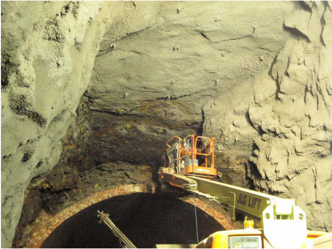
Tunnel Liner Removal in Brook Tunnel
