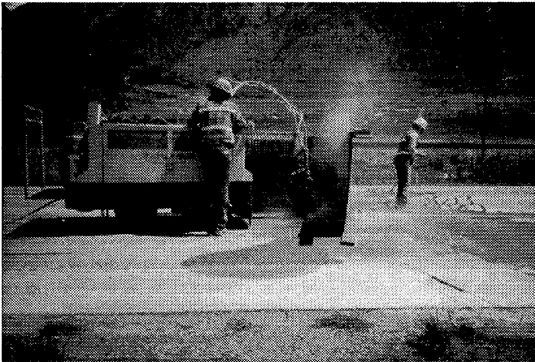
Figure 9. Waterblasting equipment with mobile robot.
