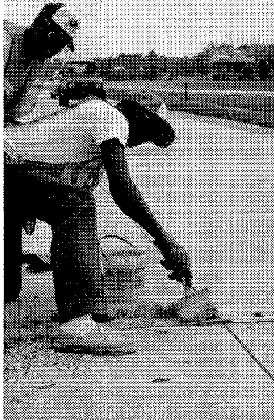
Figure 12. Application of epoxy bonding agent.
