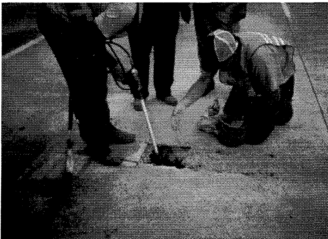
Figure 14. Placement of Percol FL.
