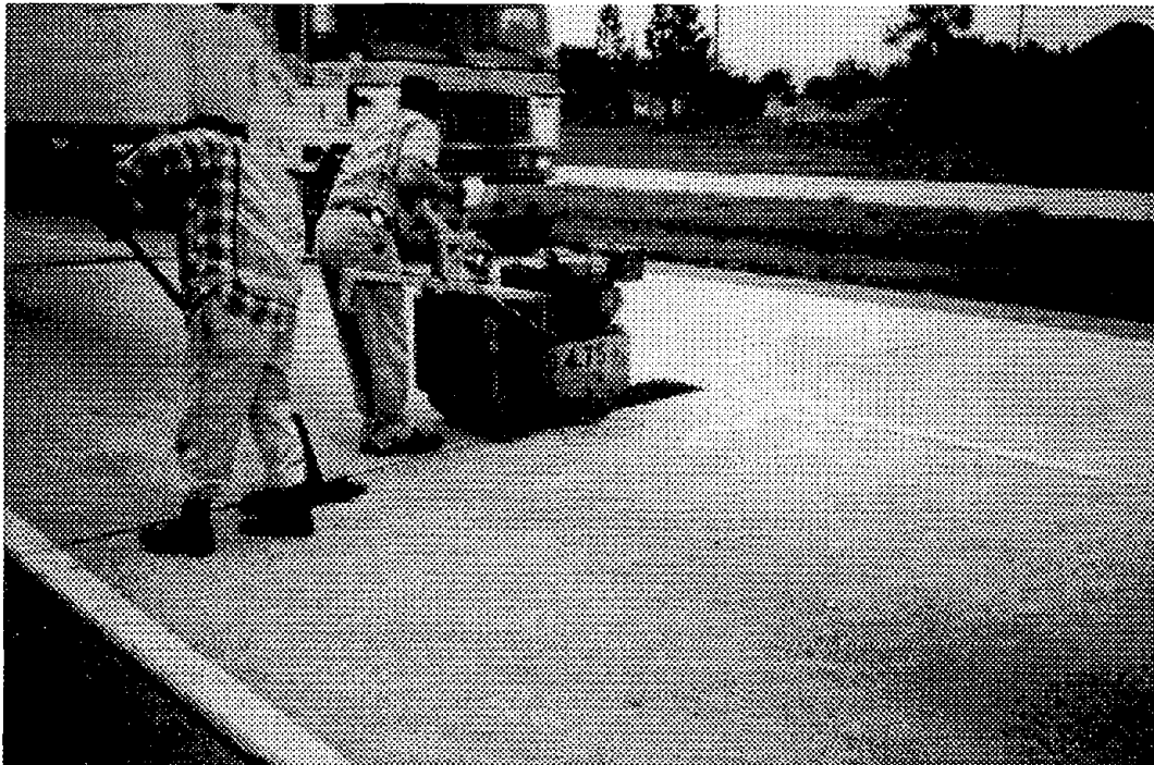
Figure 16. Compaction of UPM repair.
