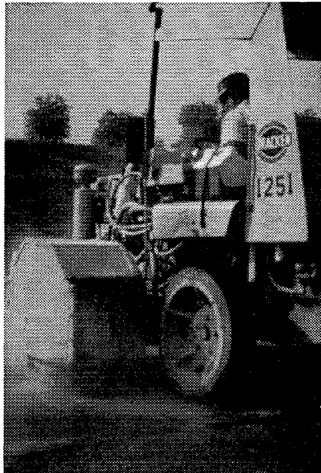
Figure 7. Carbide-tipped, cold-milling machine.
