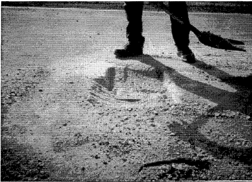
Figure 17. Patch area for milling operation.
