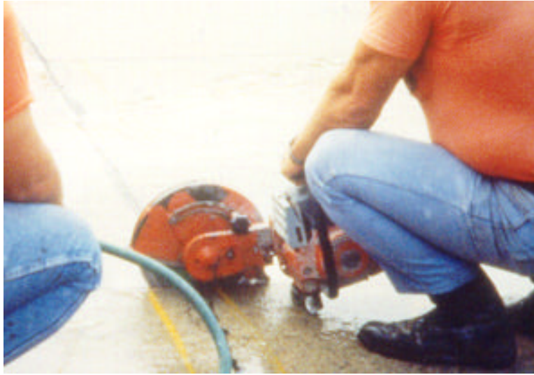
Figure 10. Sawing patch boundaries with a small handheld saw.
