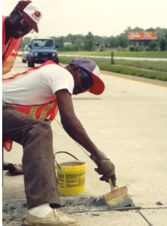
Figure 22. Applying bonding agent.
