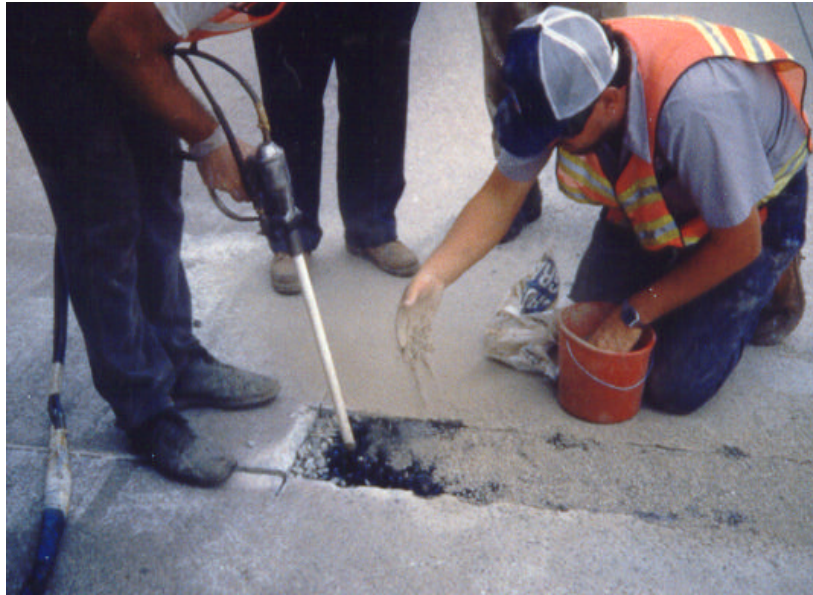
Figure 23. Pumping polymer into a patch that was prefilled with aggregate (cover aggregate also being placed).
