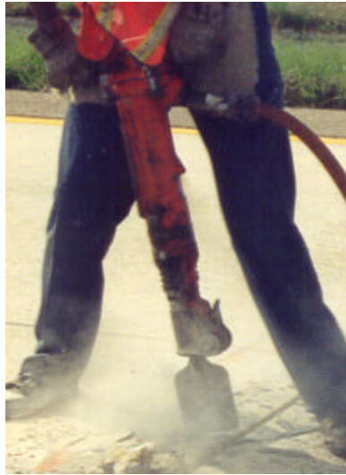
Figure 13. Using a jackhammer.
