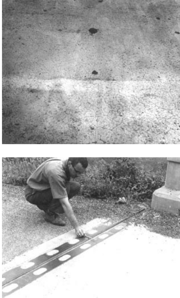
Figure 10-17 DESTRUCTIVE ALKALI-CARBONATE REACTION IN BRIDGE DECK.
