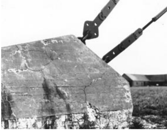
Figure 10-4 DESTRUCTIVE ALKALI-SILICA REACTION IN ANCHOR BLOCK
