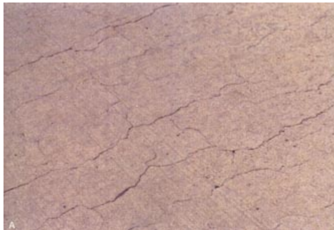
Figure 10-6 UPPER PORTION OF BACK WALL SHEARED BY EXPANSION OF BRIDGE DECK
