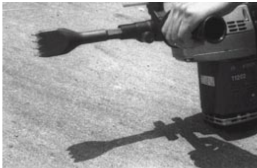
Figure 10-11 ELECTRIC HAMMER REMOVING CARBONATED SURFACE OF HCC.
