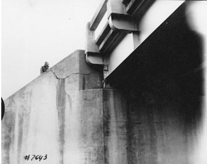
Figure 10-6 UPPER PORTION OF BACK WALL SHEARED BY EXPANSION OF BRIDGE DECK
