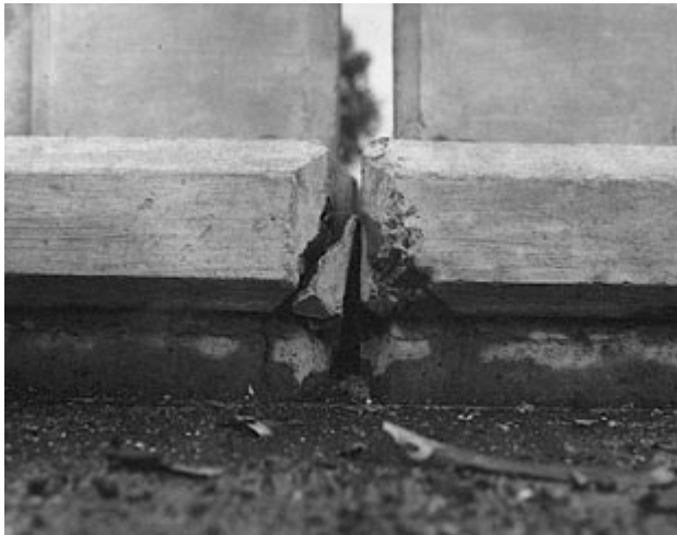
Figure 10-4 DESTRUCTIVE ALKALI-SILICA REACTION IN ANCHOR BLOCK
