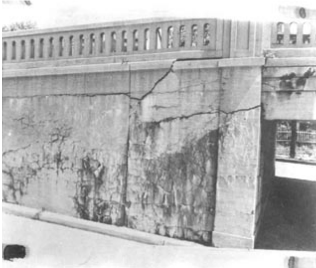
Figure 10-16 DETERIORATION DUE TO A COMBINATION ALKALI-SILICA REACTION AND ALKALI-CARBONATE REACTION. In New Jersey.
