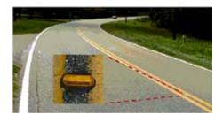
Figure. Centerline Raised-Pavement Markers.
