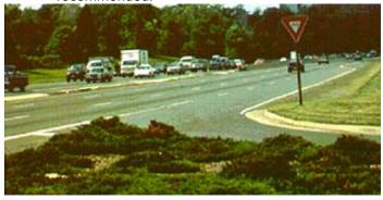
Figure. Picture of an Acceleration Lane.
