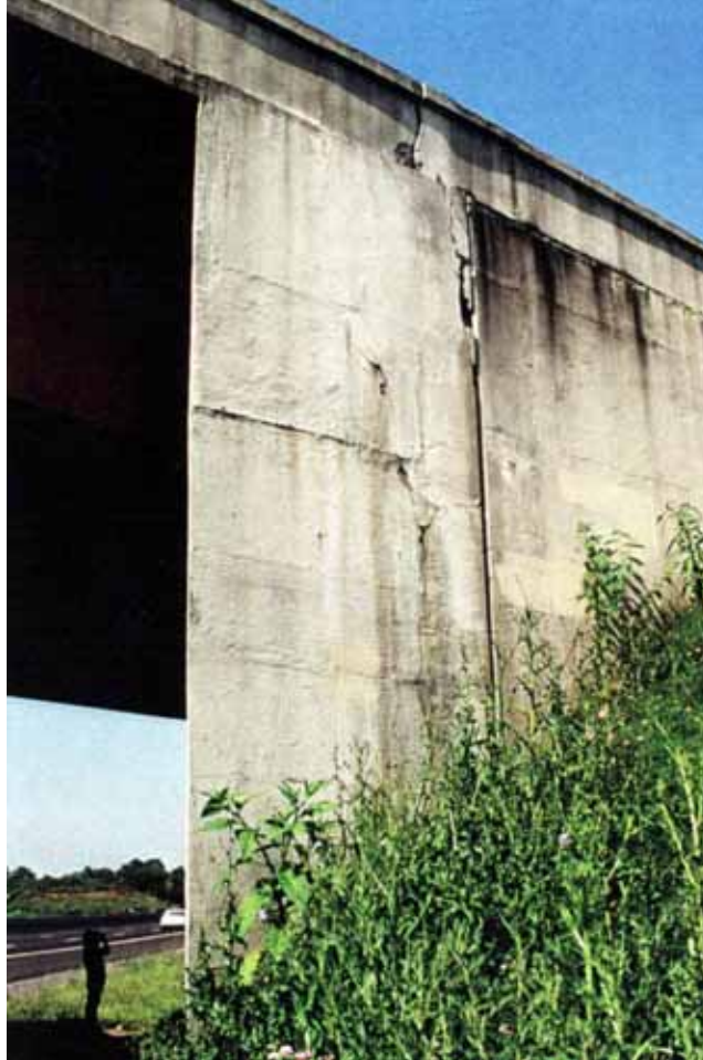
Figure 3-40. Bridge 8—north face of west abutment.
