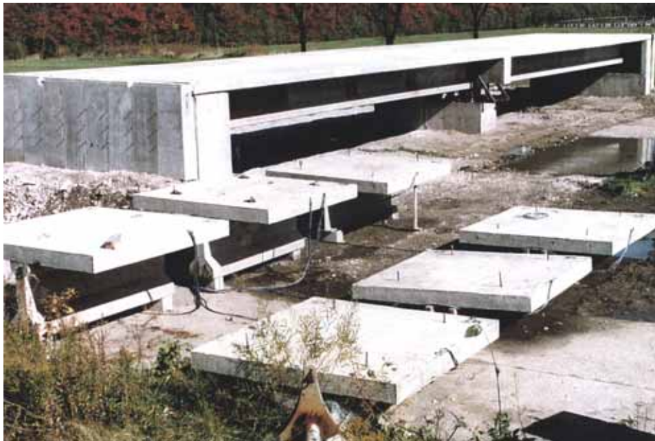
b. Slab and PS/C beam elements.
