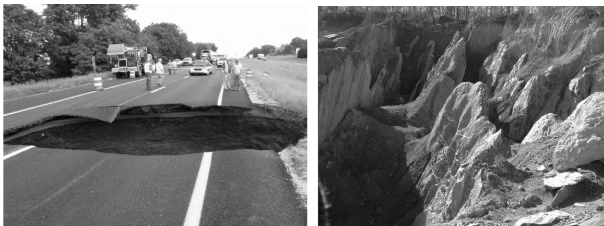
Figure 12-1 Surface expressions of karst: (a) sinkhole in Tennessee and (b) pinnacled bedrock.
