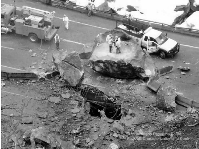
Figure 12-25 Rockfall event in Glenwood Canyon, CO affecting I-70 in 2010 (CDOT, 2017).
