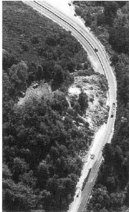
Figure 12-19 Route 17 landslide from Loma Prieta earthquake (from Kavazanjian, et al., 2011).
