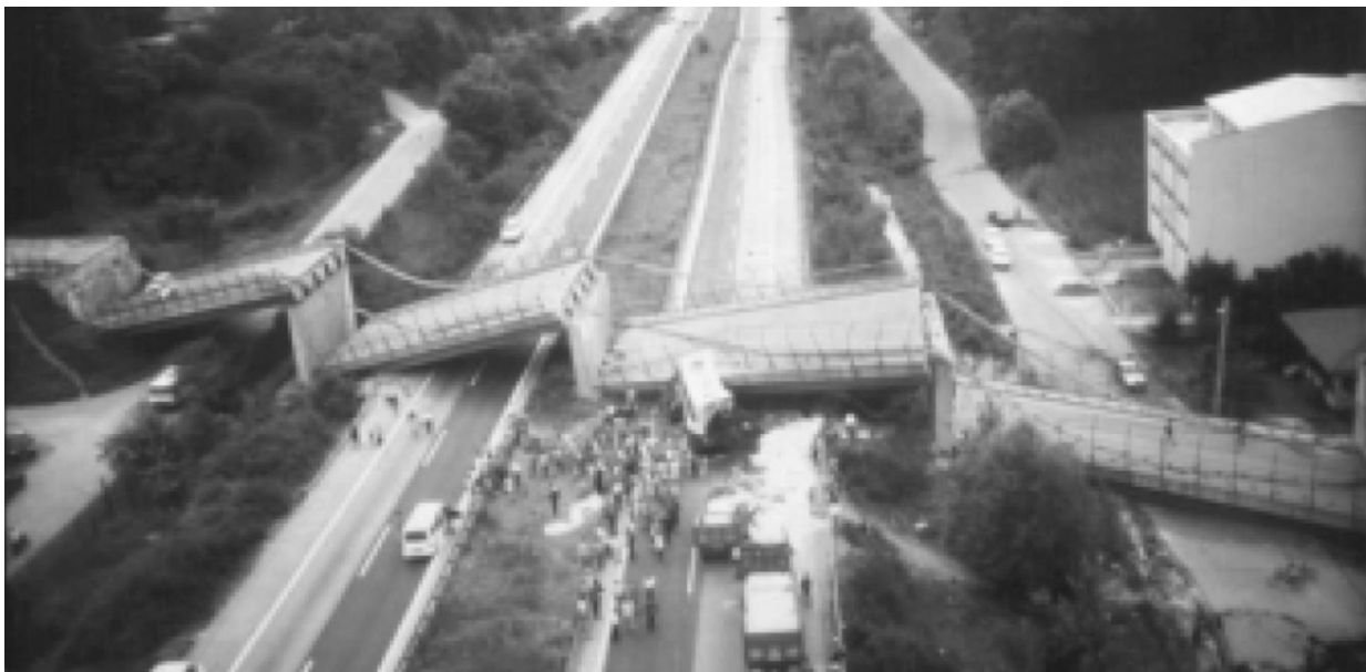
Figure 12-21 Collapse of overpass on highway in Kocaeli, Turkey earthquake (from Erdik, 2001).
