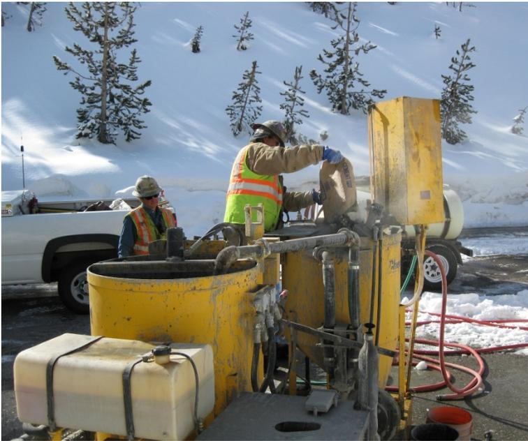
Figure 3.4: Photo. Typical grout plant setup.
