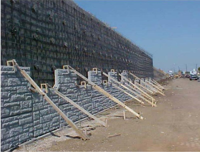
Figure 3.20: Photo. Precast panel facing. Photograph courtesy of Texas DOT.
