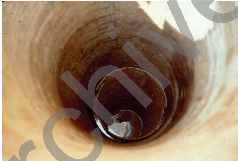
Figure 4-13 Telescoping Casing
