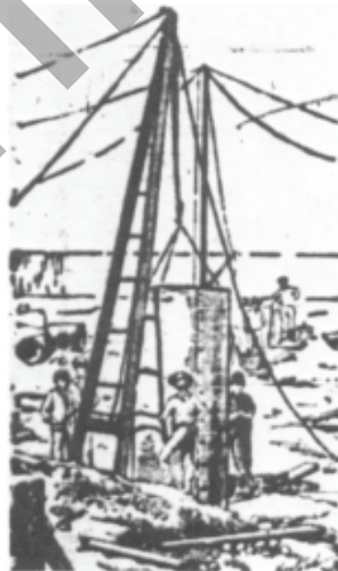
Figure 1-5 “Caisson” Foundation Construction in Kansas City (Hoffmann, 1966)
