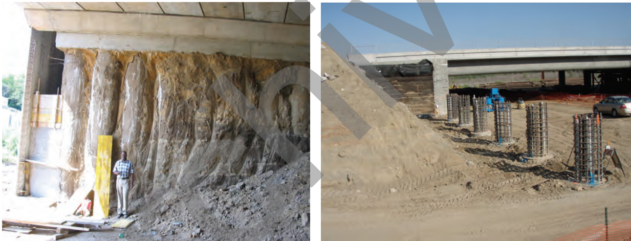
Figure 12-7 Drilled Shaft Abutment Foundations
