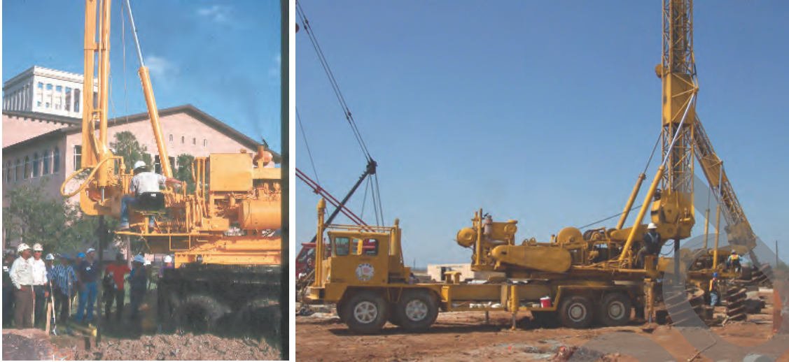
Figure 5-4 Truck Mounted Drilling Rigs
