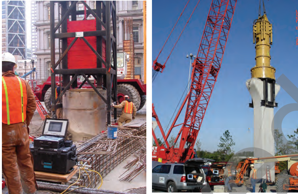
Figure 17-35 Dynamic Load Test of Drilled Shafts using Drop Weight (left) and Pile Hammer (right). [Photos courtesy of Pile Dynamics, Inc. (left) and Ross McGillivray (right)]
