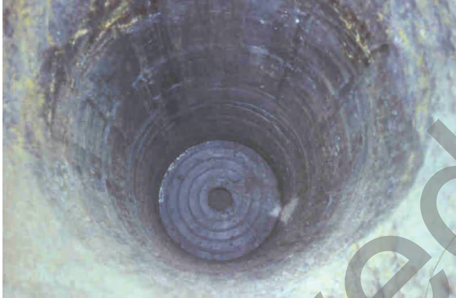
Figure 4-1 Dry Hole in Stable Soil
