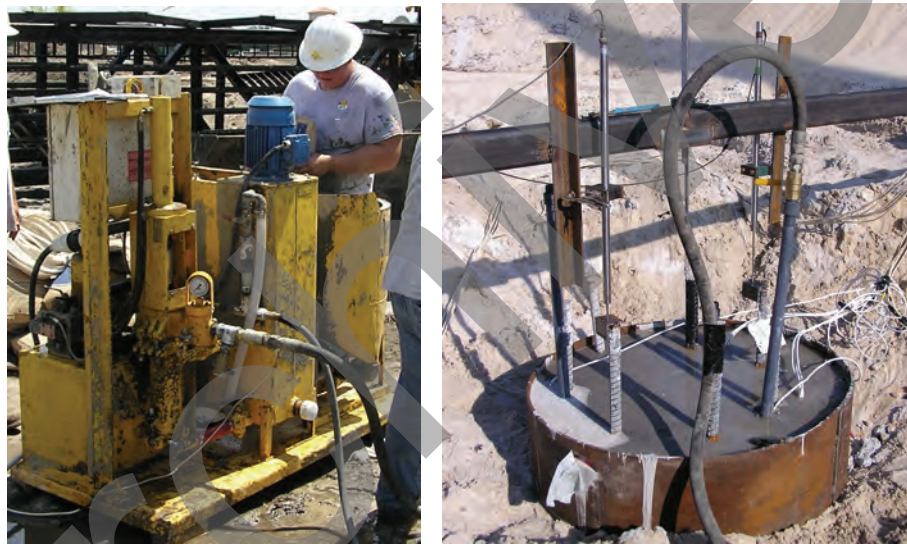
Figure 4-22 Pumping Grout to the Base of the Shaft
