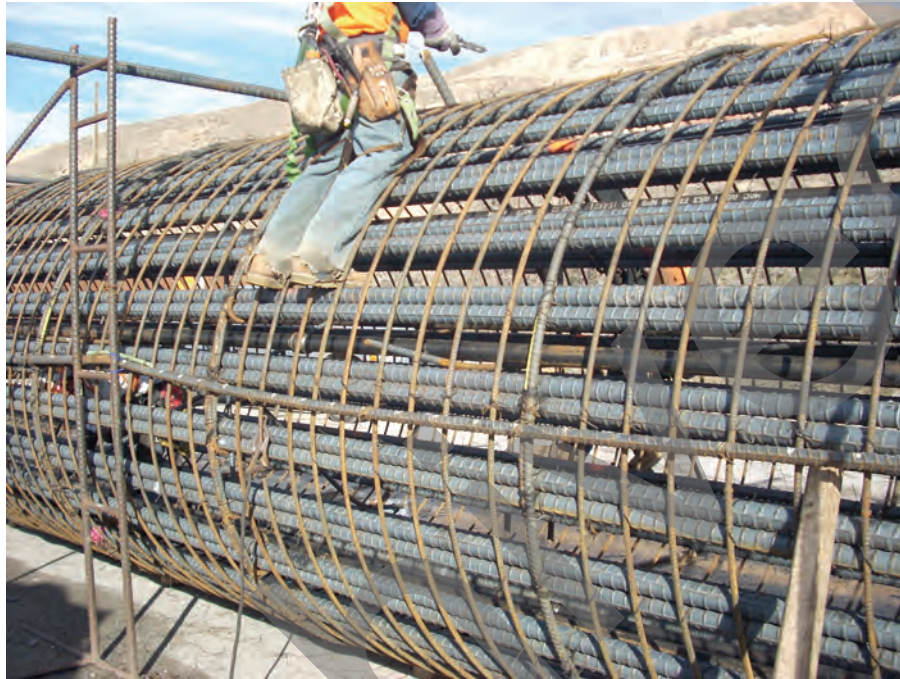
Figure 8-3 View of Bundles of No.18 Rebar in a Drilled Shaft Cage
