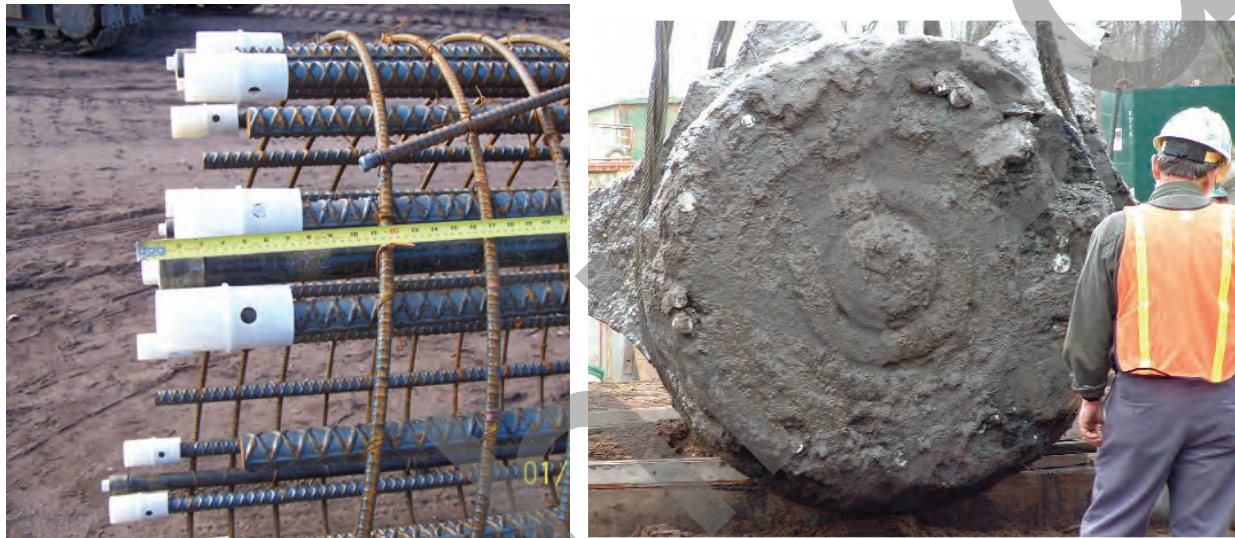
Figure 8-17 Chairs for Base of Reinforcing Cage
