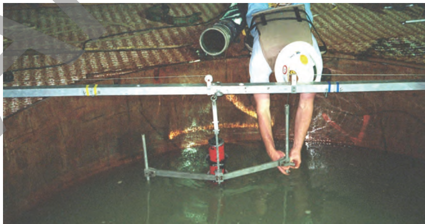
Figure 19-1 Setting Up a Sonic Caliper for Profiling a Drilled Shaft
