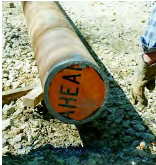
Figure 9-10 Closure Plates for Closed Tremie
