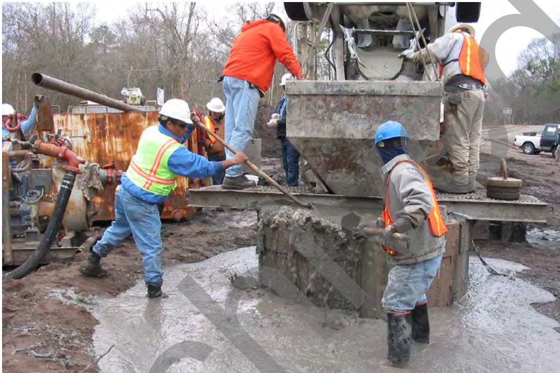
Figure 9-18 Over-pour of the Shaft Top Until Clean Concrete is Revealed
