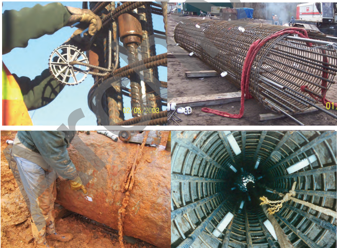
Figure 8-16 Roller Centralizers on Reinforcing Cage. Clockwise from top left: mounting external roller centralizer on the cage; completed cage with centralizers; rollers attached to hoop reinforcement; extracted shaft revealing centralizer on surface.
