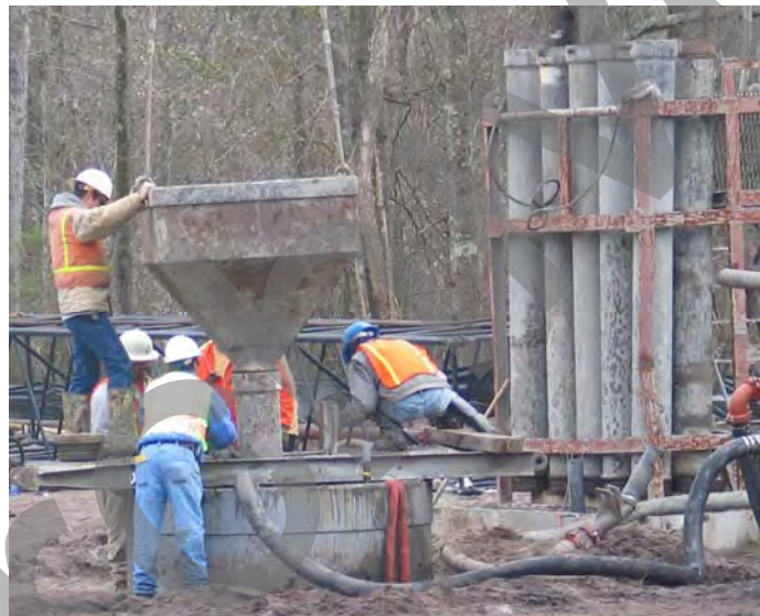
Figure 9-9 Assembly of Segmental Tremie for Concrete Placement
