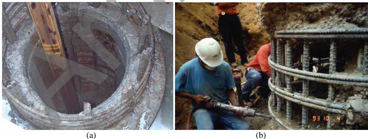
Figure 21-7 Excavation and Replacement of Defective Concrete Using (a) Drilling Tool within the Cage and (b) Hand Methods (photos courtesy Caltrans)
