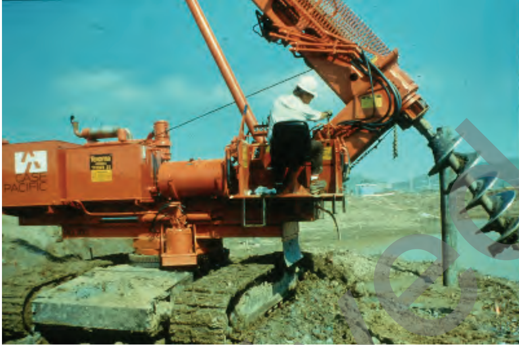
Figure 5-6 Crawler Mounted Drilling Rig
