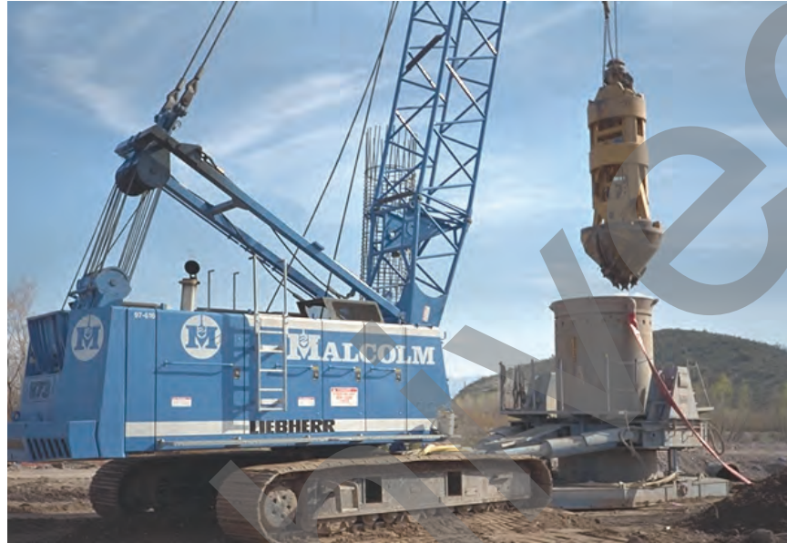
Figure 4-9 Oscillator Rig Used to Advance Segmental Casing Ahead of the Excavation
