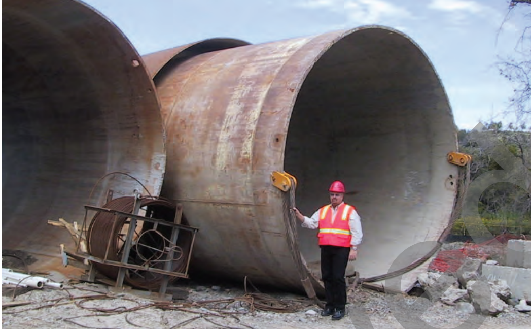
Figure 6-2 Exceptionally Large Temporary Casings
