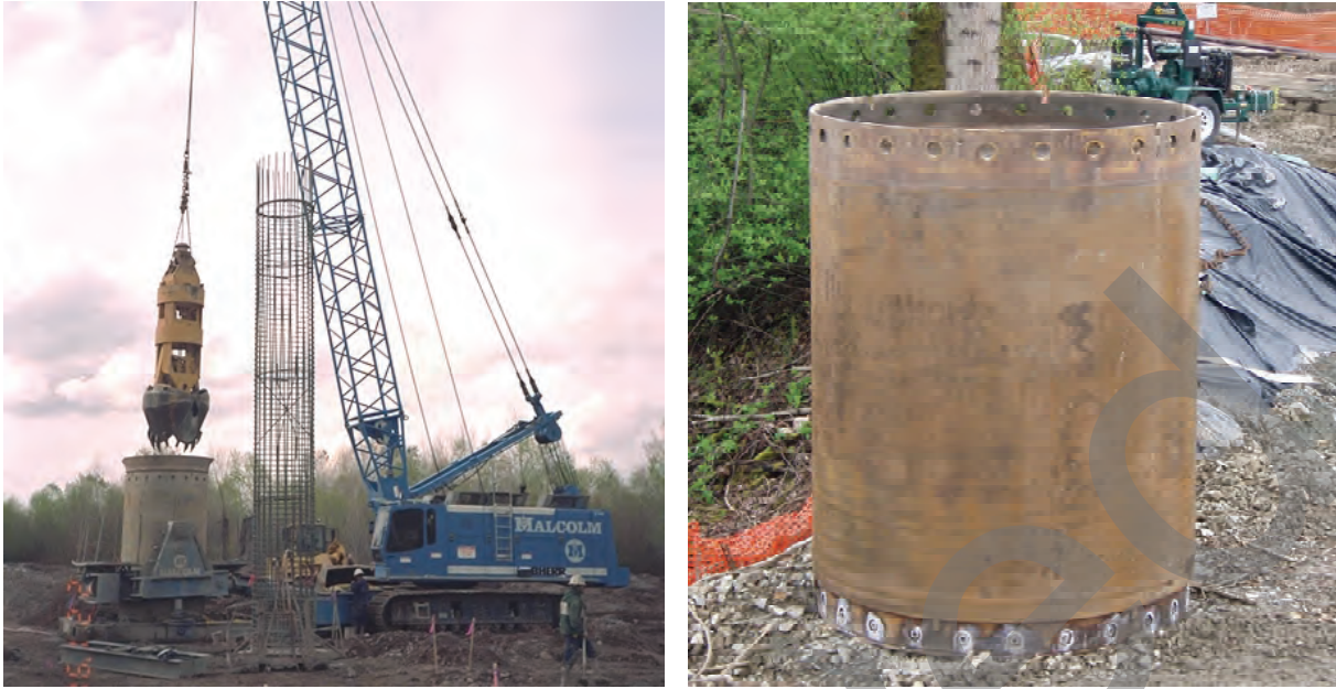
Figure 6-3 Segmental Casing Installation with Oscillator System
