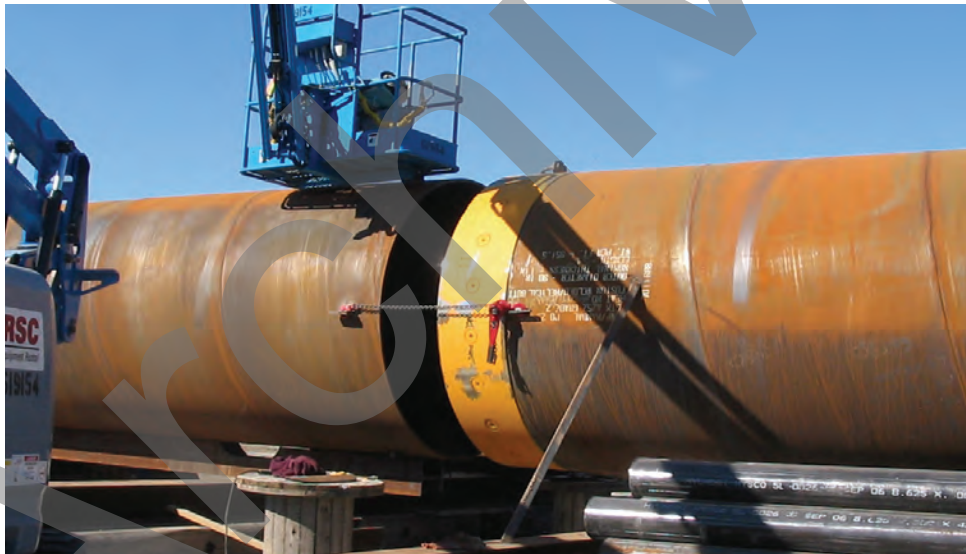
Figure 6-4 Installation of Casing Joint on Standard Pipe
