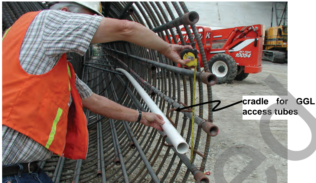
Figure 20-7 Placement of PVC Access Tube Inside Reinforcing Cage
