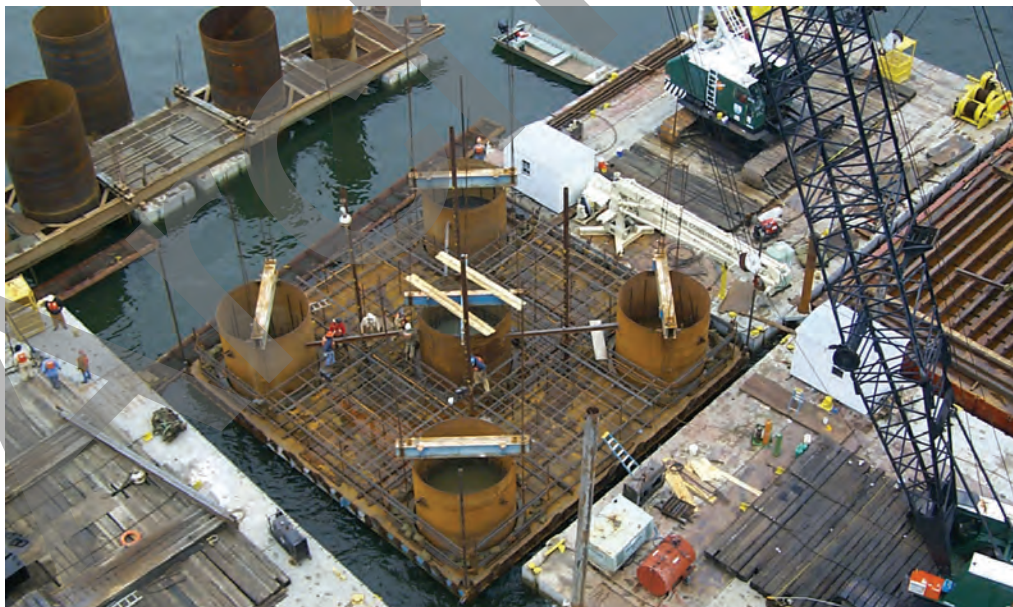
Figure 1-13 Group of Drilled Shafts for Large Loads
