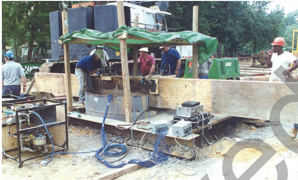
Figure 17-3 Instrumented Research Load Test
