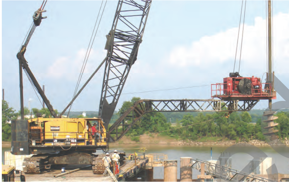
Figure 5-5 Crane Mounted Drilling Rig
