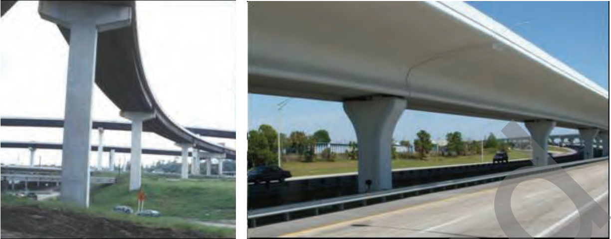
Figure 12-1 Single Column Piers with Monoshaft Foundations
