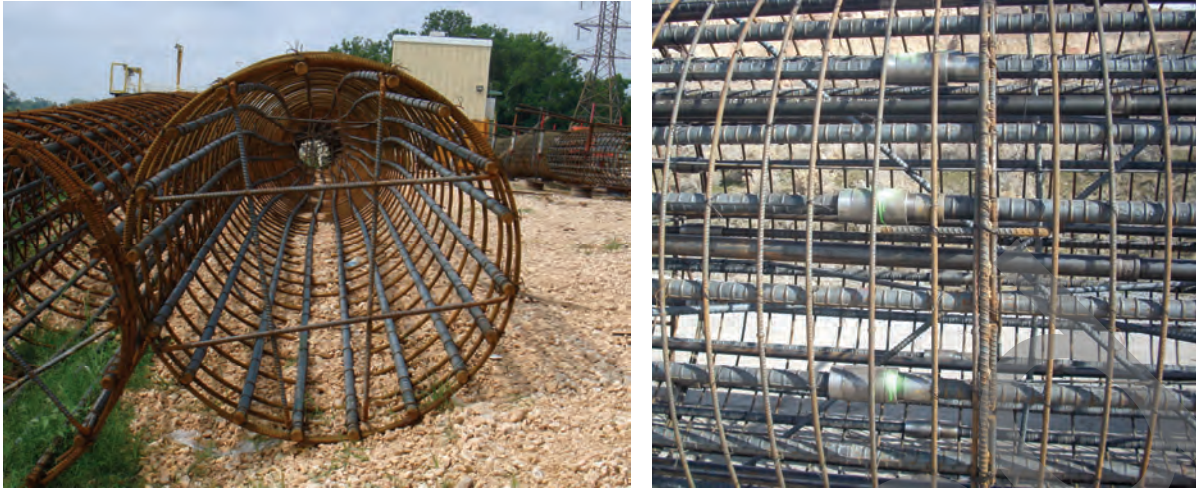
Figure 8-18 Transverse and Longitudinal Stiffeners for Temporary Strengthening of the Rebar Cage
