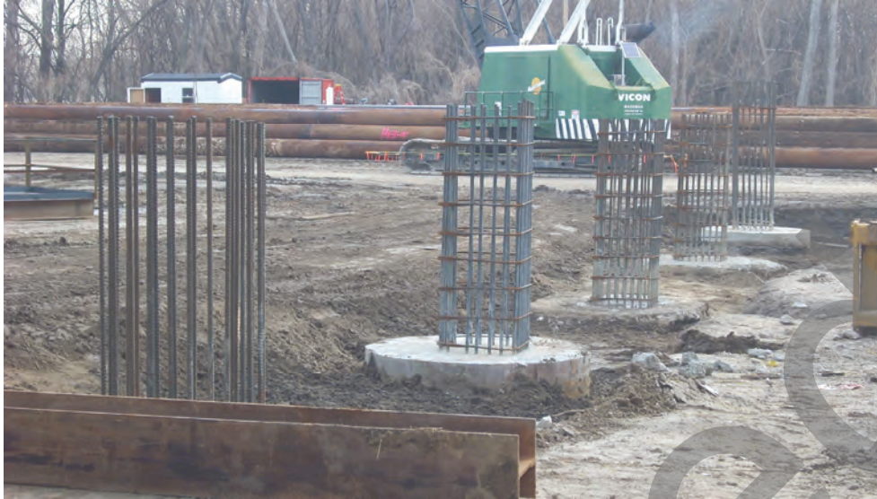
Figure 8-14 Splice Cage Used to Fabricate Column to Shaft Connection
