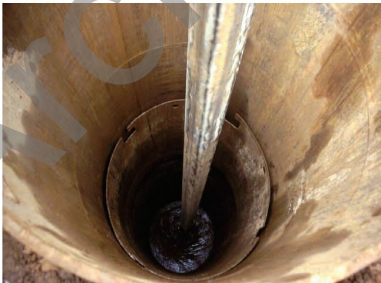
Figure 6-7 Use of Telescoping Casing
