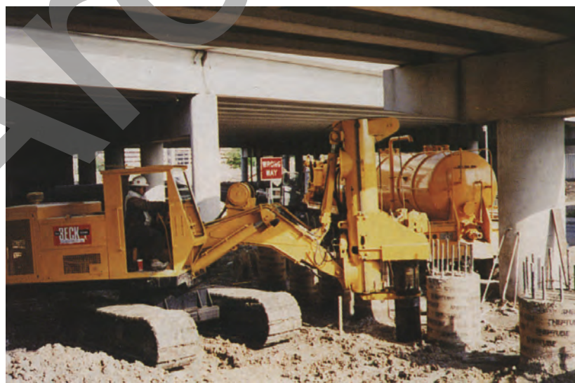
Figure 1-15 Drilled Shafts with Low Headroom
