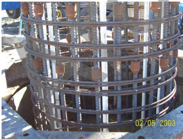
Figure 8-9 Bar Couplers Used to Construct Splices
