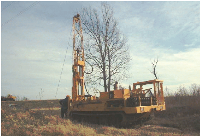
Figure 12-1. Track-Mounted Drill Rig Investigating Bridge Site in Hayti, Missouri.
