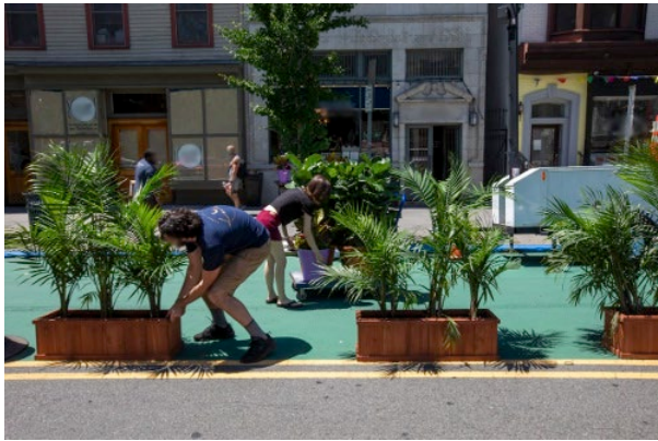
© 2024 Jersey City Department of Infrastructure. C. Adding shrubs to parking lane.
