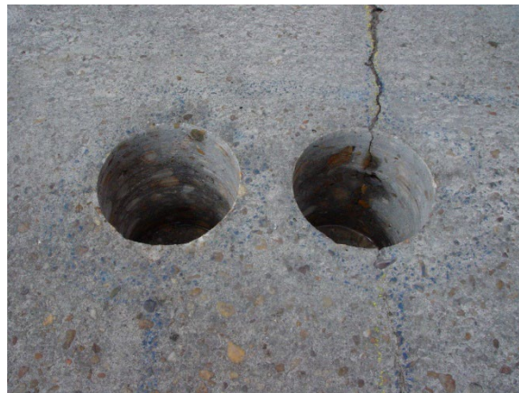
Figure 3. Photo. Cracking observed at a core hole in a concrete bridge deck during a research study on crack influence on corrosion.
