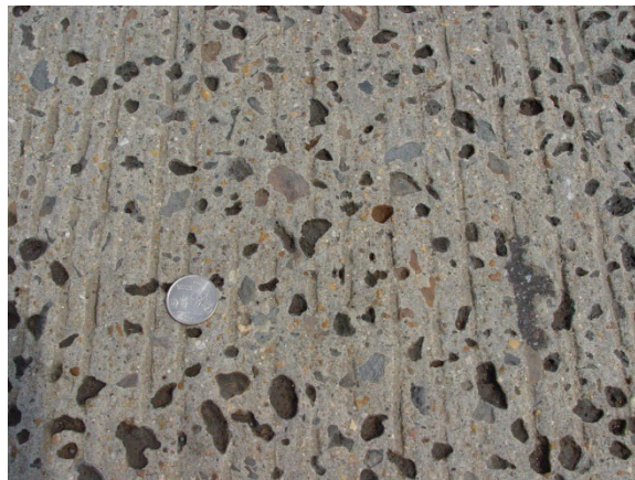
Figure 10. Photo. Degraded aggregate and cement paste loss on lightweight concrete deck.
