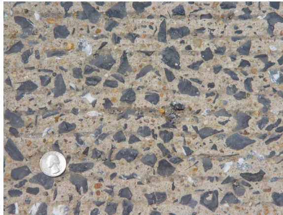
Figure 14. Photo. Loss of cement paste and polishing of aggregate on a bridge deck.
