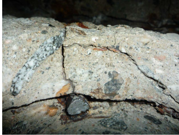
Figure 5. Photo. Extensive cracks caused by the corrosion of reinforcing steel.
