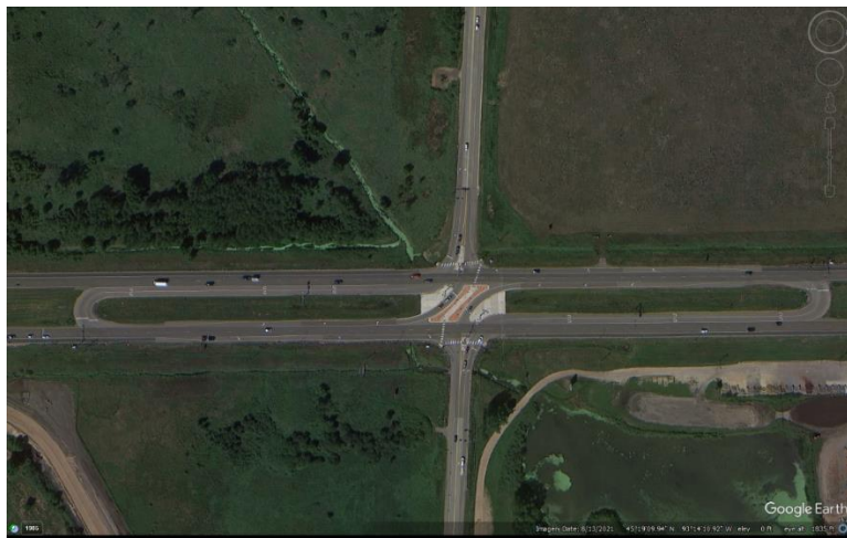
Figure 22. Photo. MN-65 at Viking Avenue intersection, before condition in East Bethel, MN. (32)
