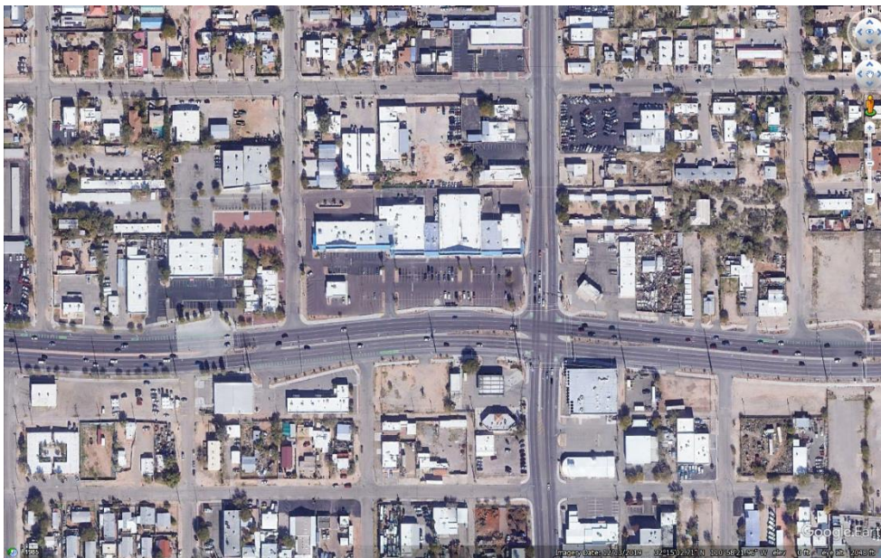
Figure 5. Photo. Grant Road at Stone Avenue intersection before condition (photo date February 23, 2017) in Tucson, AZ. (32)
