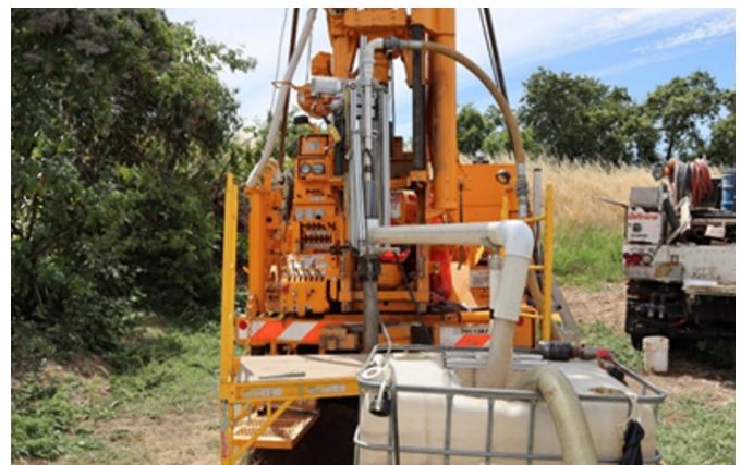
■ The ISTD equipment assembled in front of the drill rig.
