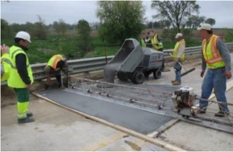
Figure 2. The installation of UHPC on the Laporte Road Bridge in 2016.
