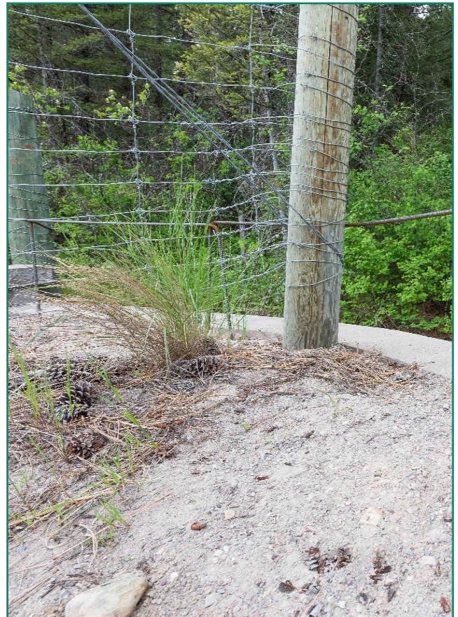
Courtesy of NDOT Research Division. One example of the researched wildlife crossing technologies in this TPF study includes an animal jump-out on U.S. Route 93 in Montana.
