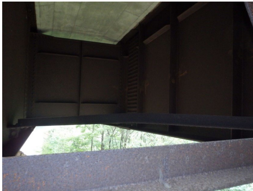
Figure 68. Photo. Out-of-plane buckling of the lower chord brace. 17
