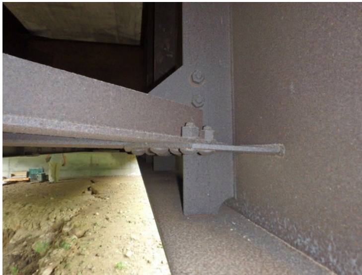
Figure 74. Photo. Undamaged connection detail for lower chord bracing. 19
