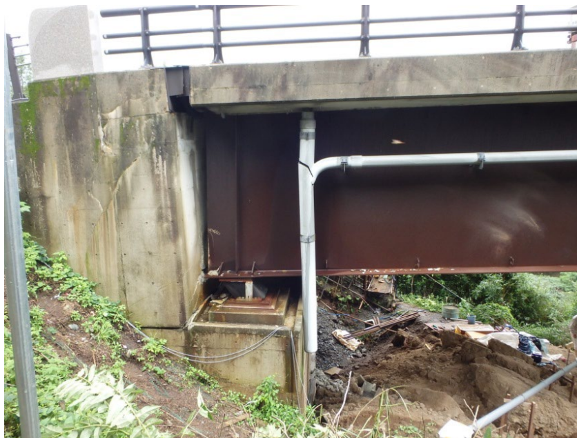
Figure 61. Photo. Failure of the west approach.
