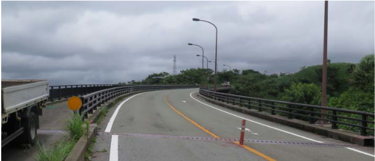
Figure 75. Photo. Ooginosaka bridge from the south approach showing left lateral offset at the abutment.
