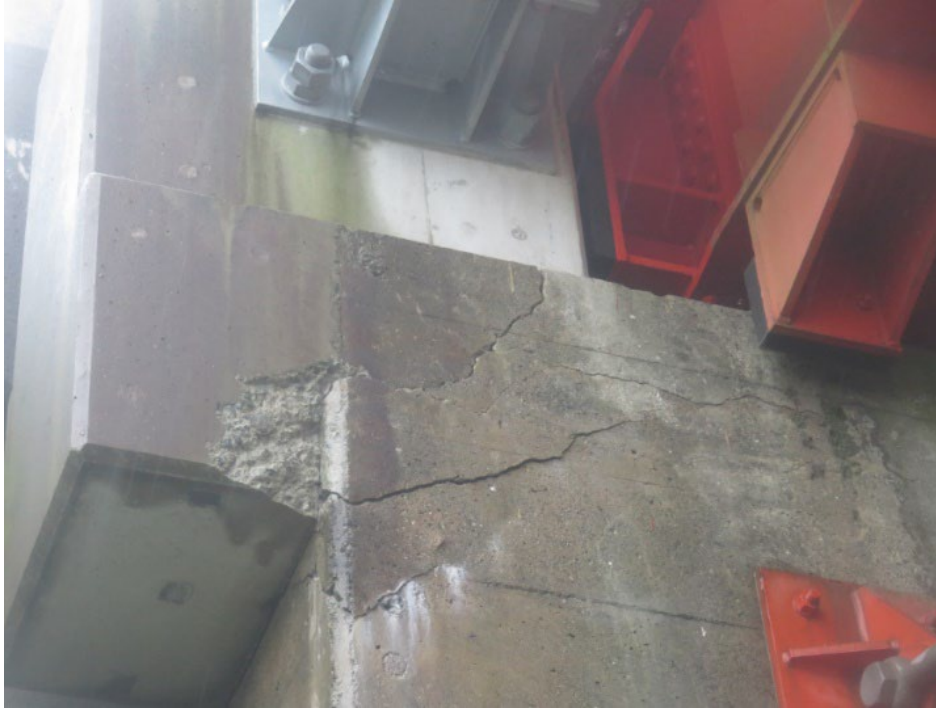
Figure 89. Photo. Damage to the shear key block on the west side of the north abutment.
