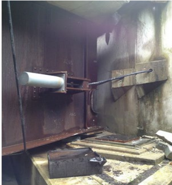
Figure 30. Photo. Failed bearing below girder G1 at abutment A2.
