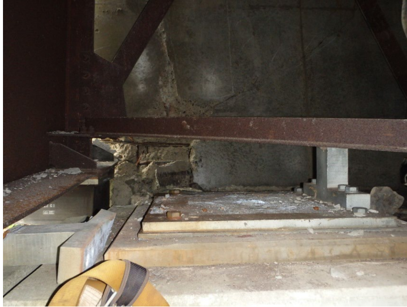
Figure 67. Photo. Failure of a bearing stopper at the east abutment. 16
