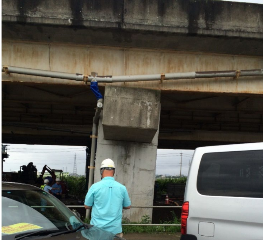
Figure 95. Photo. Side view of tilted pier P11.
