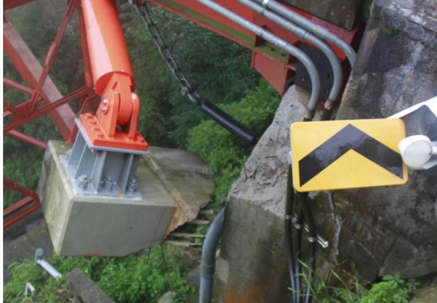
Figure 85. Photo. Damage to the anchorage of longitudinal damper and shear key on the west side of the south abutment.
