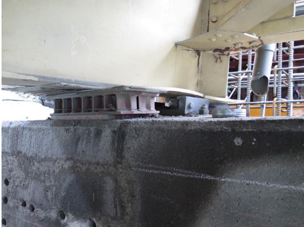
Figure 106. Photo. Damaged expansion bearing and girder at abutment A1.
