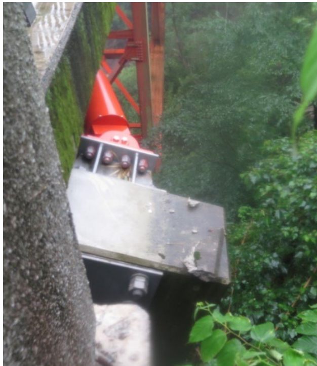
Figure 86. Photo. Damage to the anchorage of the longitudinal damper and shear key on the east side of the south abutment.
