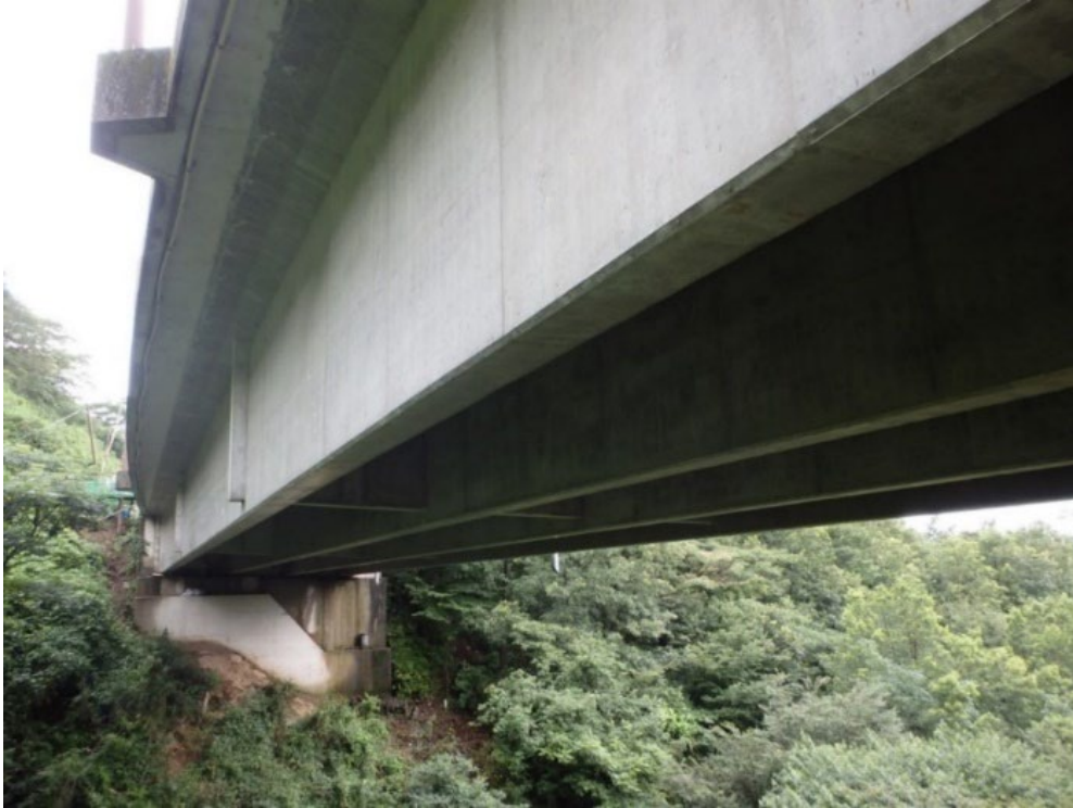
Figure 50. Photo. Susukinohara bridge showing concrete T-girder superstructure with diaphragms. 8
