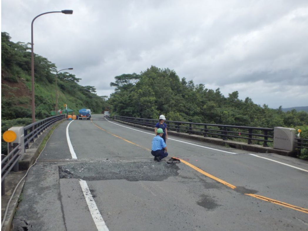
Figure 51. Photo. Distant view of damaged approach at the west abutment. 9
