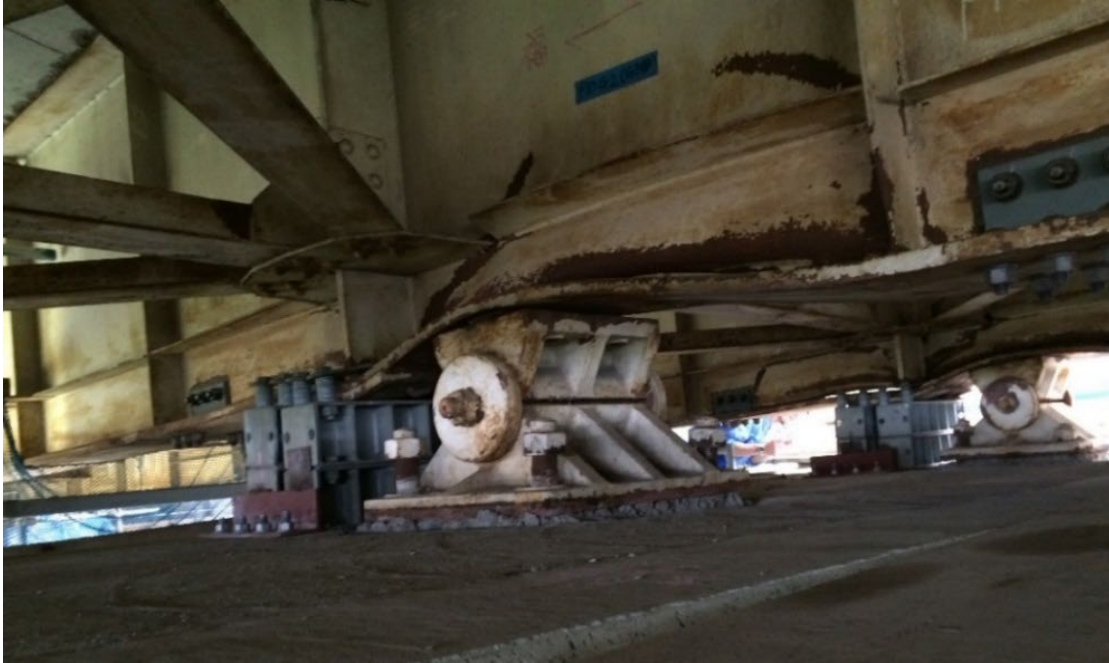
Figure 100. Photo. Failed bearing connections under interior girders at pier P10 of the east bridge.
