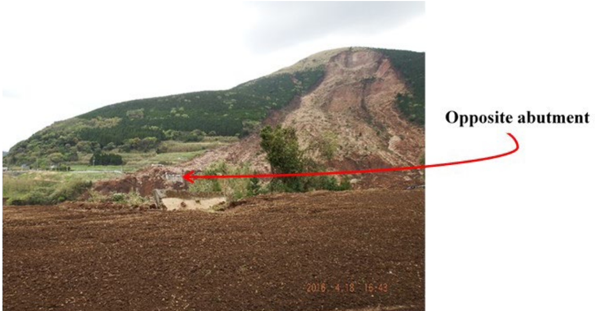
Figure 124. Photo. Landslide upstream of the west abutment across the gorge causing bridge collapse. 31
