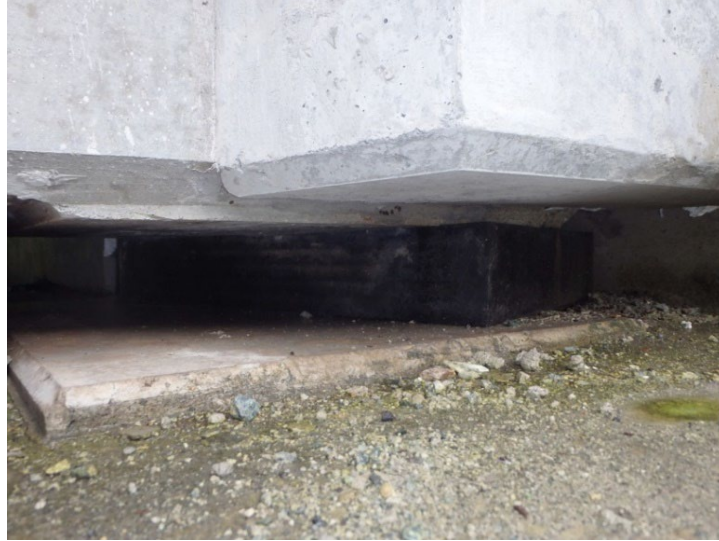
Figure 54. Photo. Rotation of an elastomeric bearing. 10
