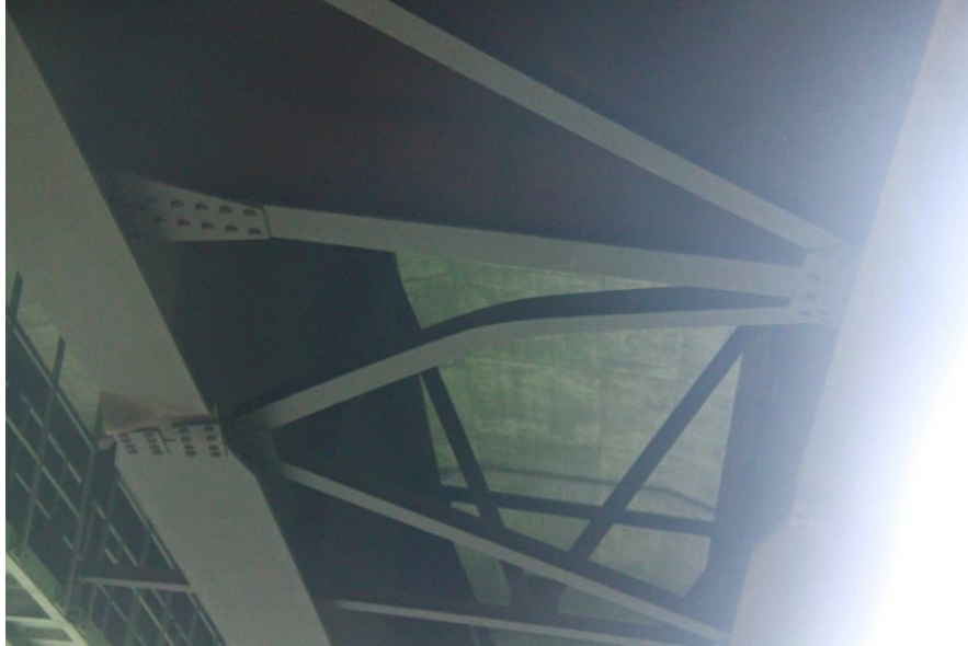
Figure 69. Photo. In-plane buckling of lower chord braces.
