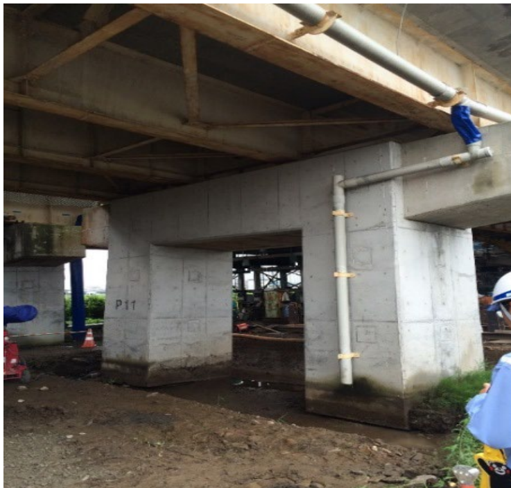
Figure 95. Photo. Side view of tilted pier P11.
