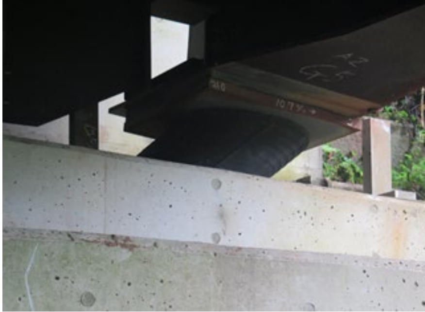
Figure 77. Photo. North abutment with easterly superstructure shift.
