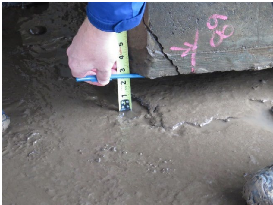
Figure 96. Photos. Exposed column-to-pile cap connection at pier P11 of the east bridge.
