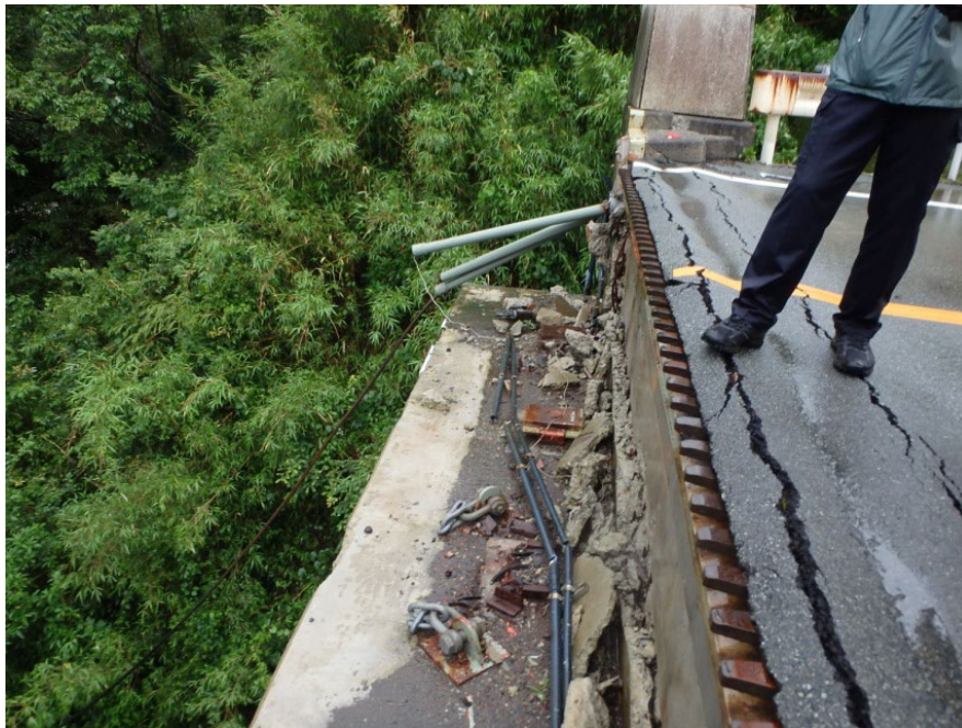
Figure 122. Photo. Unseated first span below the east abutment. 29
