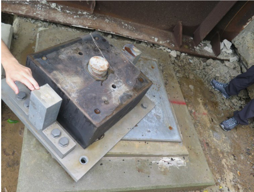
Figure 71. Photo. Elastomeric bearing and transverse stopper at the east abutment showing rotation of the bearing and implied bolt fractures in anchor plates.
