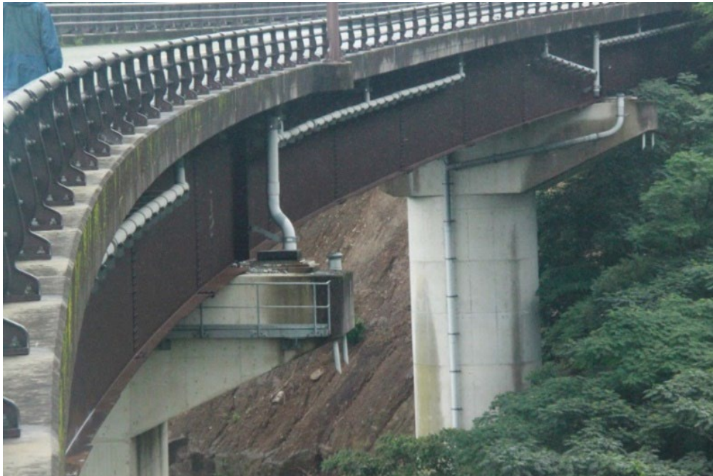
Figure 25. Photo. Offset of superstructure at piers P3 and P4.
