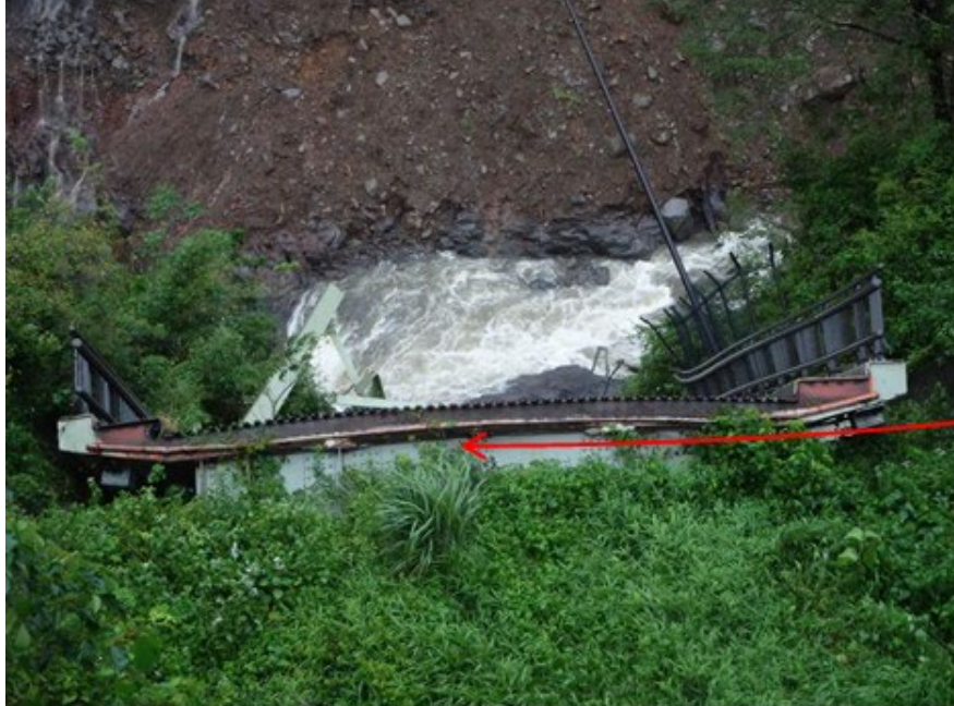
Figure 122. Photo. Unseated first span below the east abutment. 29
