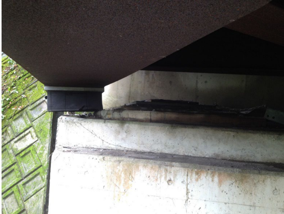
Figure 30. Photo. Failed bearing below girder G1 at abutment A2.
