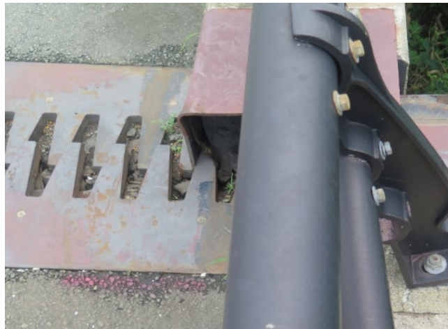
Figure 76. Photo. Finger joint relocking.
