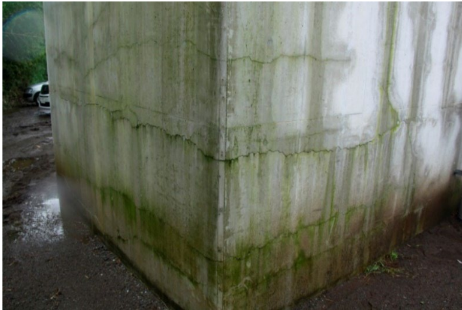
Figure 28. Photo. Cracks at the base of pier P2.
