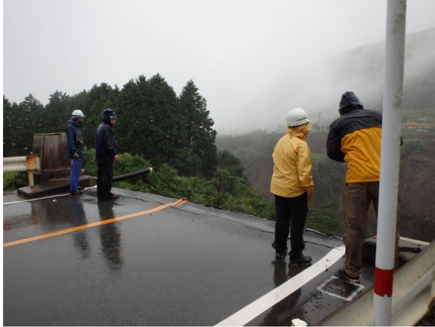
Figure 120. Photo. Remainder of the approach slab at the east abutment.
