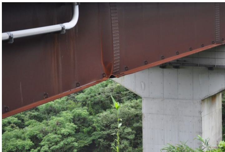
Figure 64. Photo. Buckled girder flange and web.
