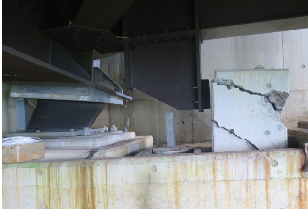
Figure 83. Photo. South abutment shear key damage.
