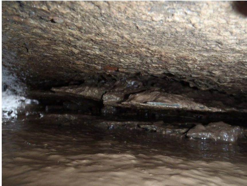
Figure 98. Photo. View into the gap at the column-pile cap connection at pier P11 of the east bridge.
