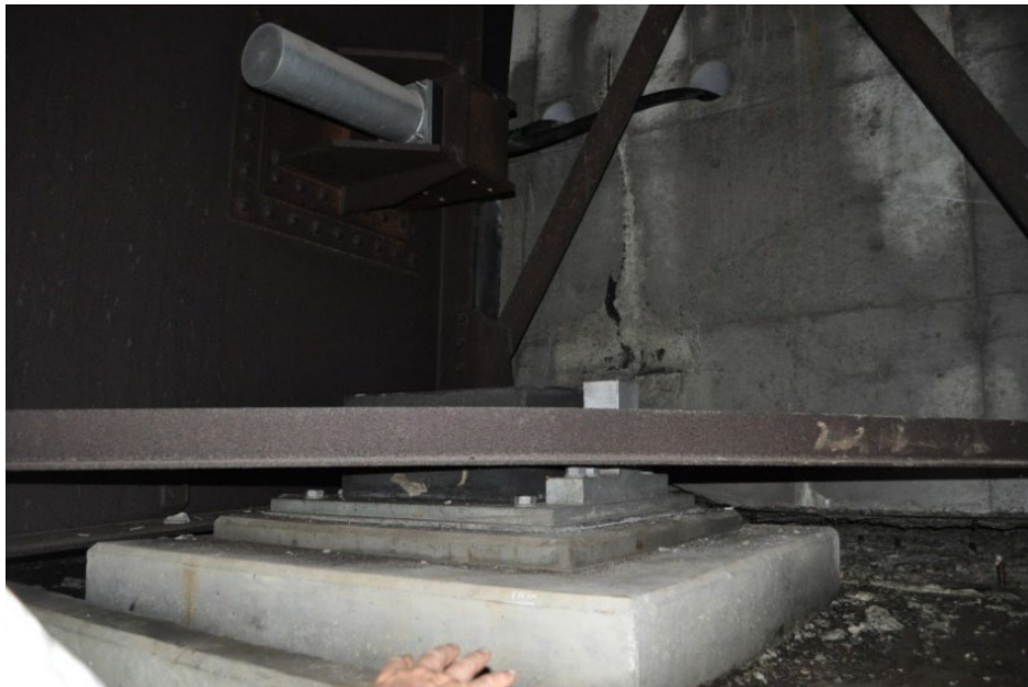
Figure 70. Photo. Longitudinal restrainer unable to prevent girder unseating transversely, as might be expected.
