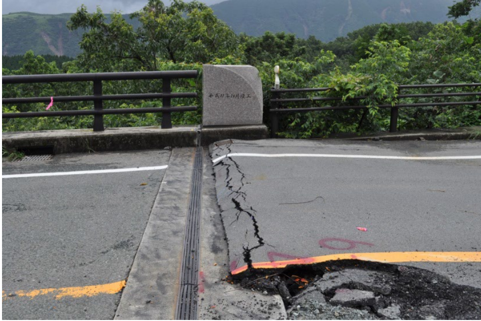
Figure 52. Photo. Close-up view of damaged approach at the west abutment.
