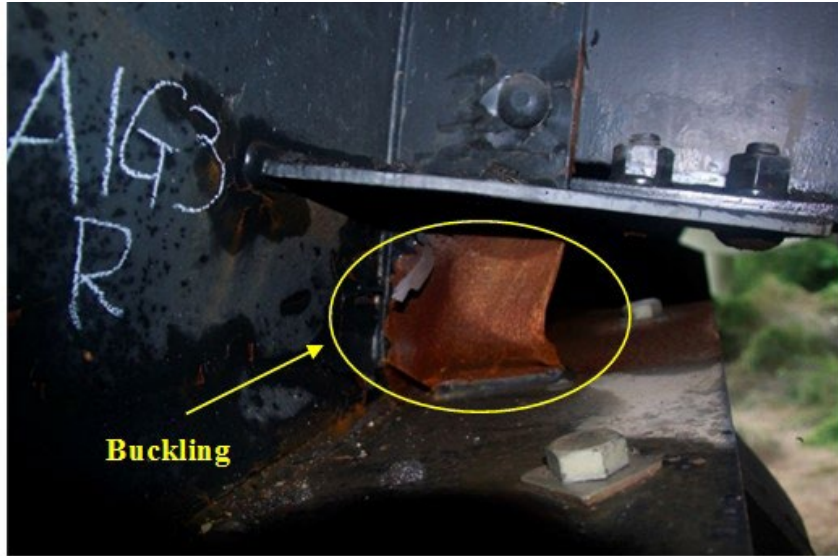
Figure 24. Photo. Damage in girder-to-diaphragm connection at abutment A1.
