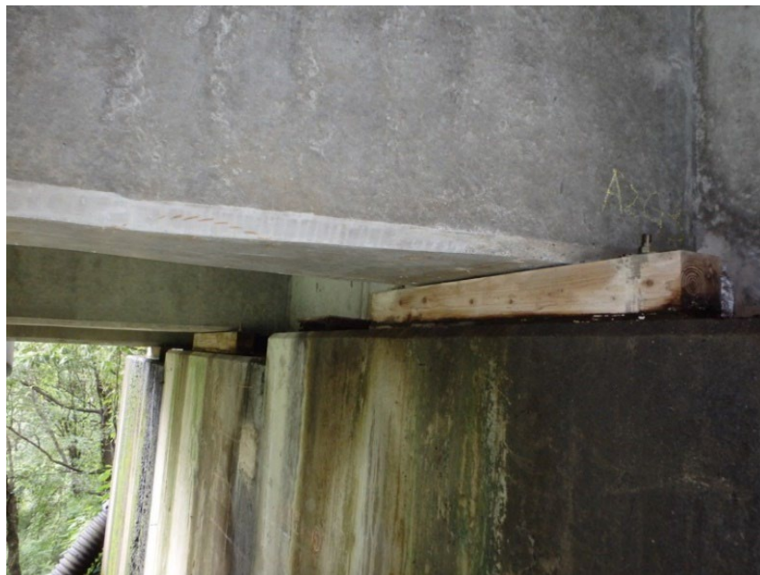
Figure 54. Photo. Rotation of an elastomeric bearing. 10
