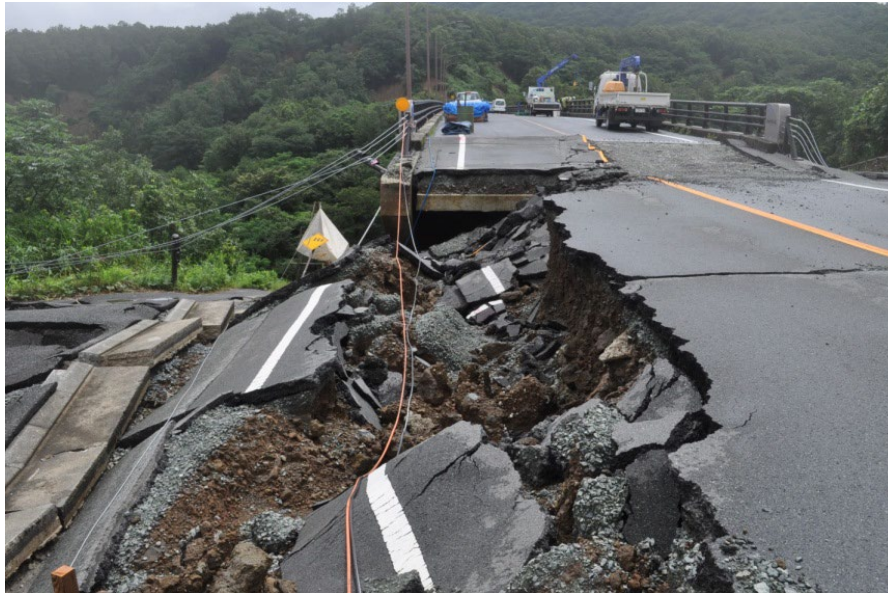
Figure 61. Photo. Failure of the west approach.
