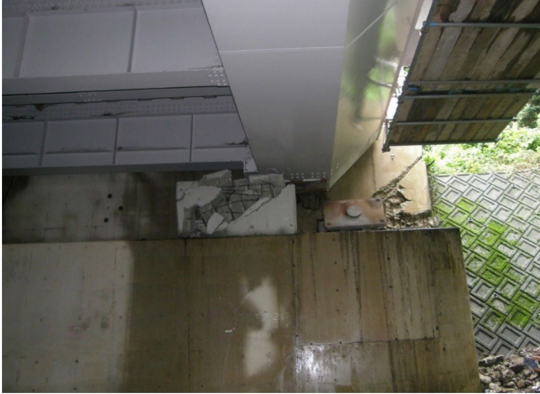
Figure 41. Photo. Damage to steel bearings at abutment A2.
