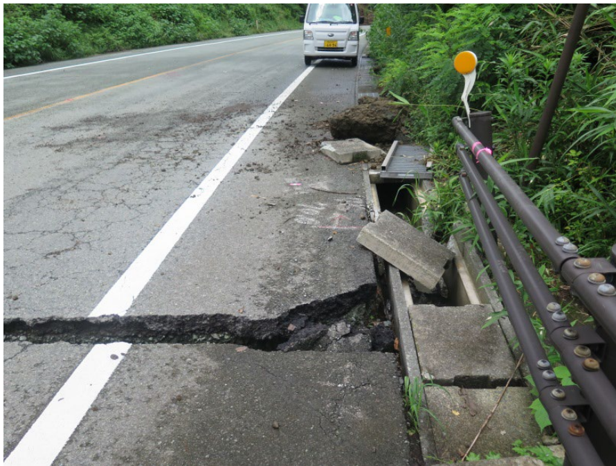
Figure 52. Photo. Close-up view of damaged approach at the west abutment.
