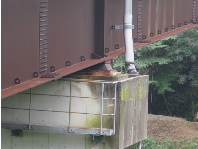
Figure 72. Photo. Permanent deformation in the elastomeric bearing on pier P1.
