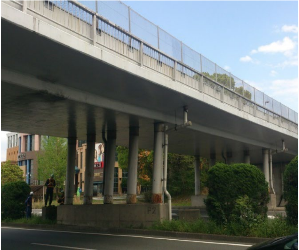
A. Inclined columns after the earthquake.
