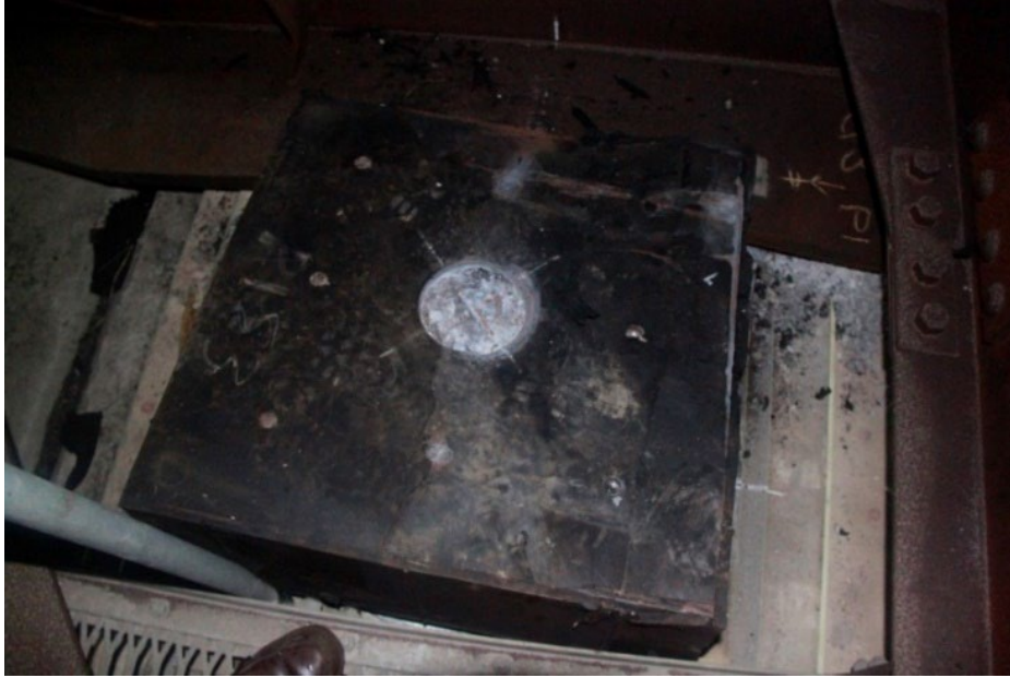
Figure 27. Photo. Elastomeric bearing at pier P1.
