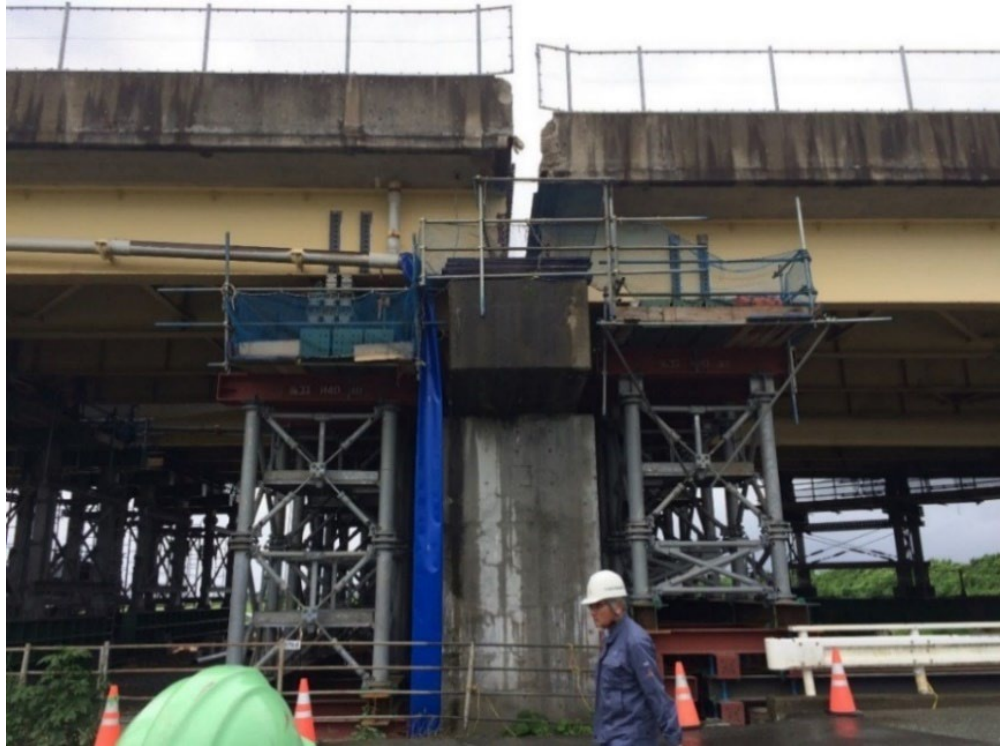
Figure 92. Photo. Opening of the expansion joint at pier P12 of the east bridge.
