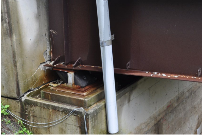
Figure 63. Photo. Pounding at the west abutment and permanent bearing deformation.
