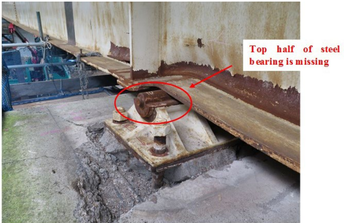
Figure 100. Photo. Failed bearing connections under interior girders at pier P10 of the east bridge.
