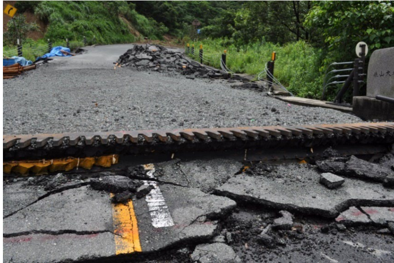
Figure 65. Photo. Vertical offset at the east abutment between the bridge and approach pavement.
