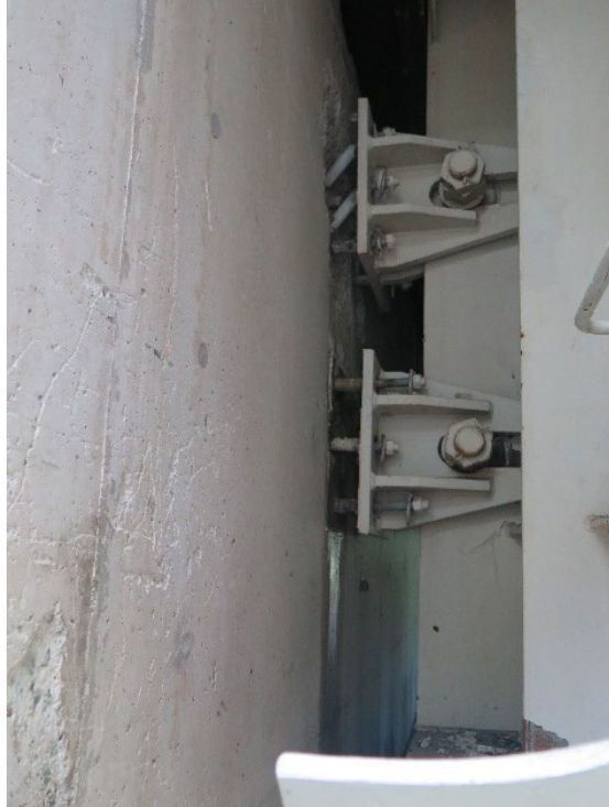
Figure 39. Photo. Damaged restrainers at abutment A1.
