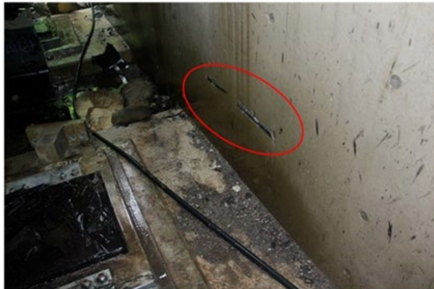
Figure 23. Photo. Abrasion on the back wall of abutment A1.
