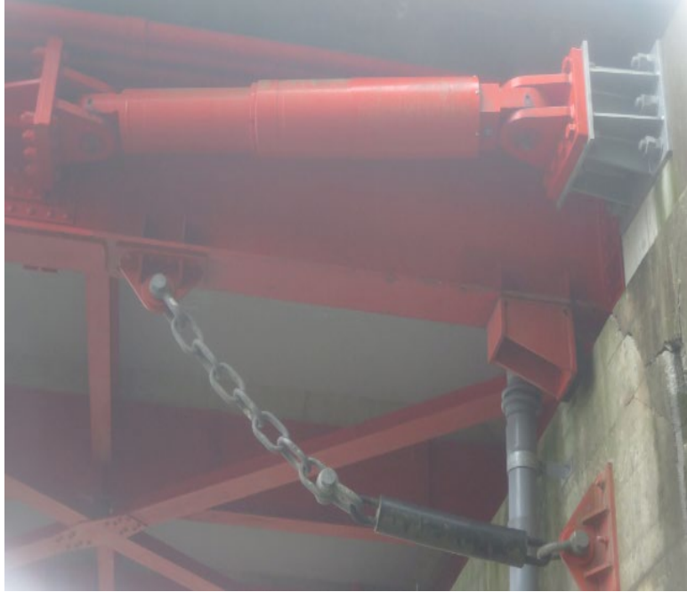
Figure 87. Photo. Longitudinal damper on the east side of the north abutment.
