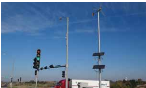
Roadway Wind/Solar Hybrid Power Generation and Distribution System (RHPS) in place.
