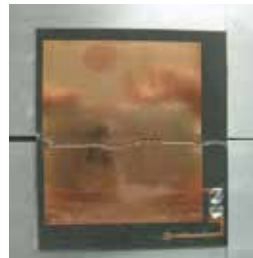
Antenna sensor tracking crack propagation.
