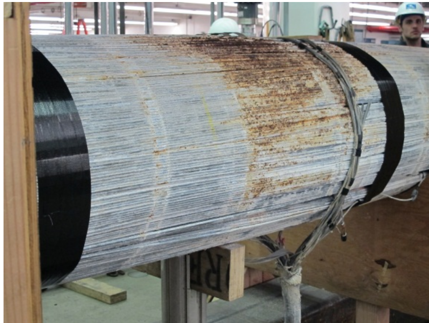
Figure 130. Photo. Corroded area under neoprene wrapping.
