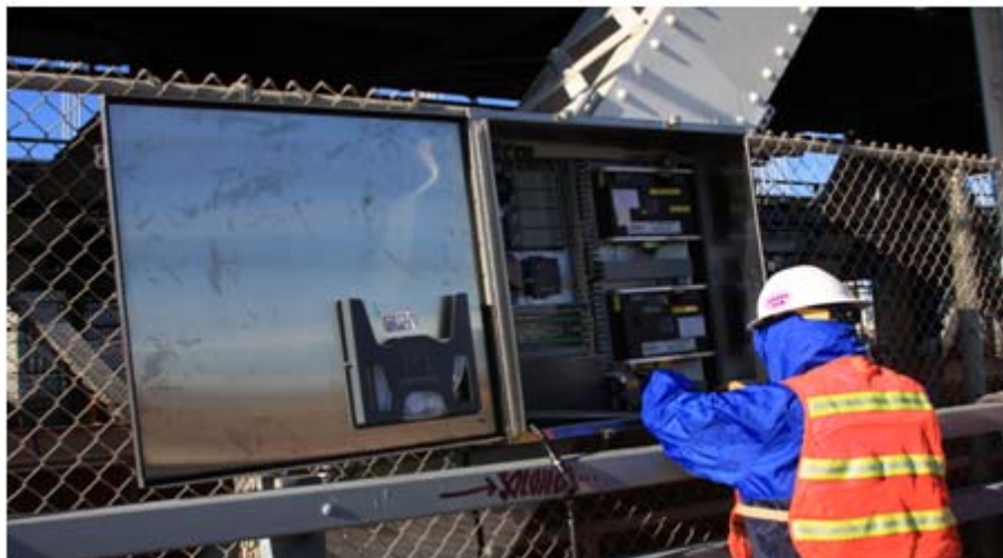
Figure 200. Photo. Installation of the central DAQ system.
