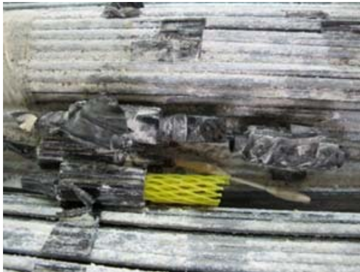
Figure 166. Photo. LPR sensor 6 during cable disassembly.
