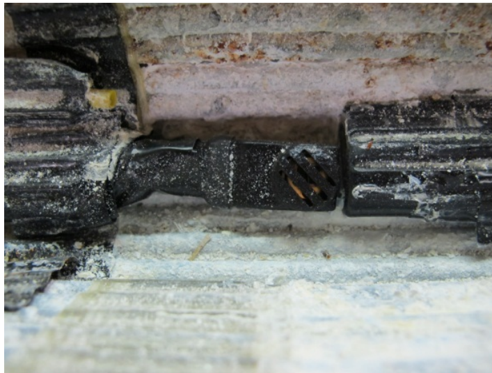
Figure 160. Photo. Close-up view of Precon HS2000V sensor 13 electrode.
