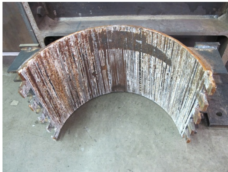
Figure 142. Photo. Interior of top of south side of cable band.
