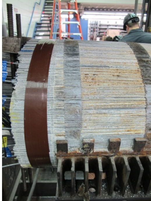
Figure 137. Photo. North end of cable with band removed.
