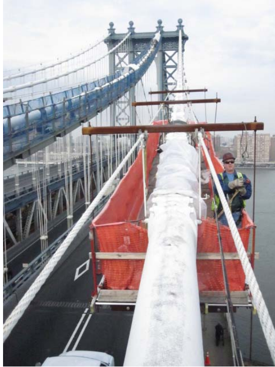
Figure 190. Photo. Suspended platform between panel points 13 and 15.
