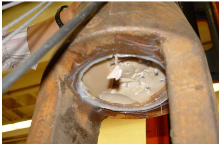
Figure 48. Photo. Failure of the epoxy filler inside the sockets.
