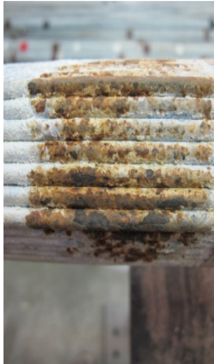
Figure 150. Photo. Close-up view of the wires with stage 4 corrosion.
