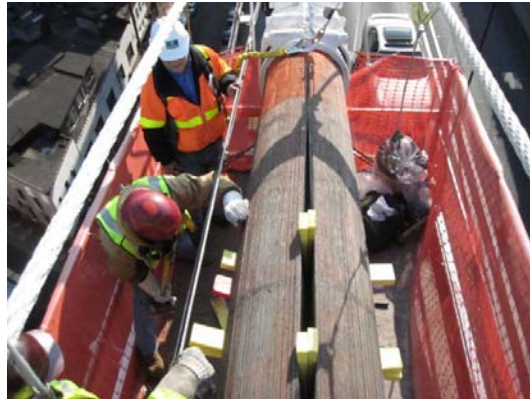
Figure 192. Photo. Cable preparation by unwrapping and wedging.
