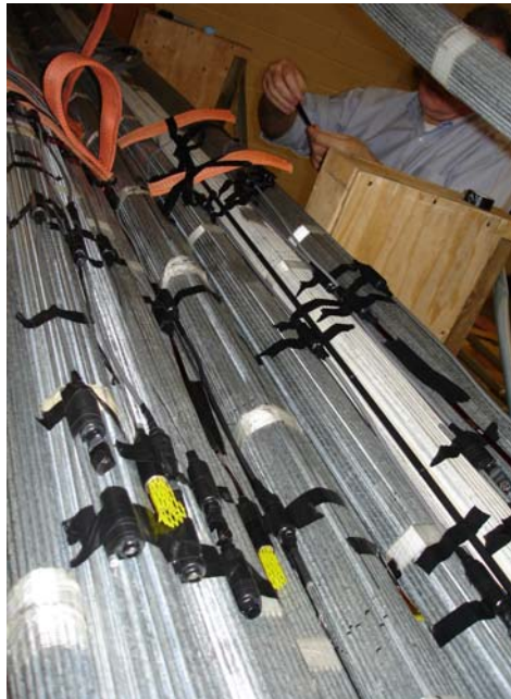
Figure 81. Photo. Placement of sensors inside the cable mockup.
