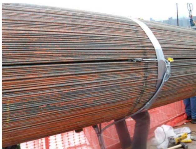
Figure 196. Photo. Sensor lead wires exiting from the cable after installation.
