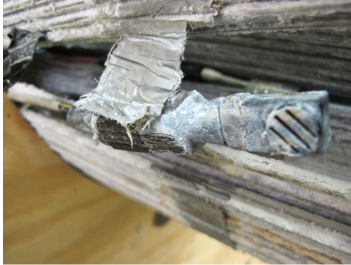
Figure 161. Photo. Precon HS2000V sensor 7 close-up of electrode during cable dissection.
