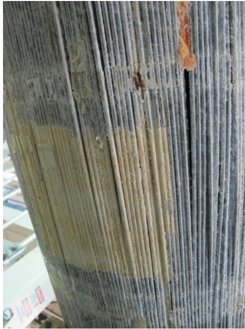
Figure 145. Photo. Product that formed where the 11.89-by-11.89-inch (30.5-by-30.5-cm) hole was placed in the aluminum cable cover.
