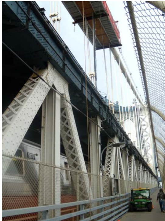
Figure 191. Photo. Walkway where the DAQ was installed.
