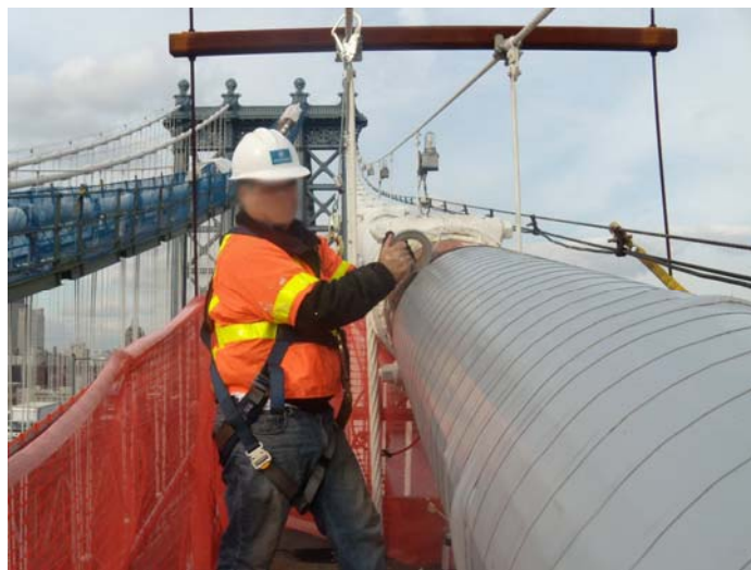
Figure 198. Photo. Final stage of the installation of the neoprene wrapping.
