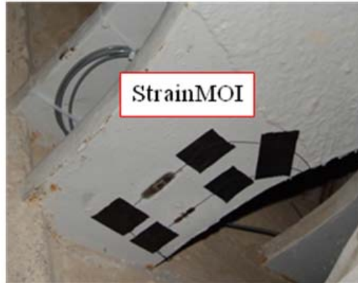
Figure 186. Photo. Strain gauges mounted on the eyebar.
