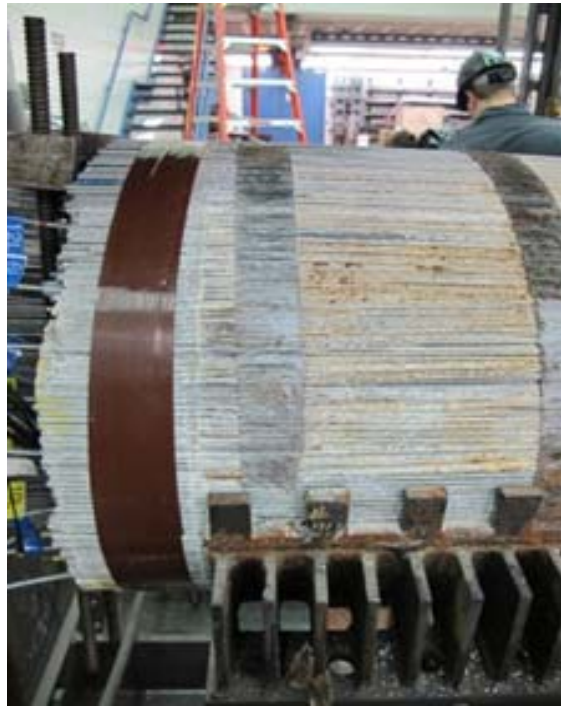
Figure 126. Photo. North side cable end following cable band removal.
