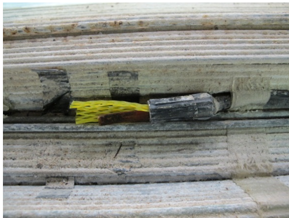
Figure 170. Photo. LPR sensor 8 during cable dissection.
