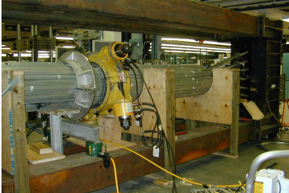
Figure 82. Photo. Cable compaction.
