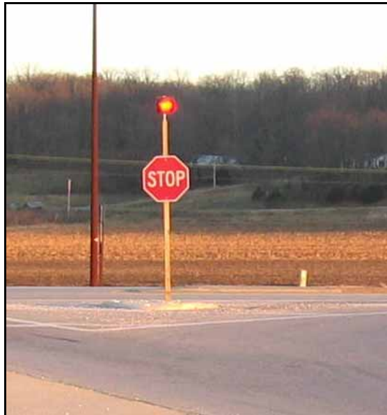
Figure 2. Photo. Example of a STOP Sign Mounted Flashing Beacon.
