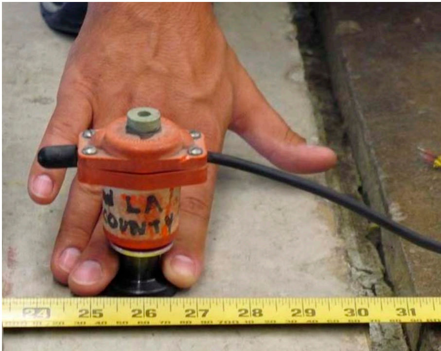
Figure 39. Photo. Locating a place to install the ball-joint floor anchor.
