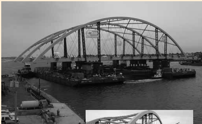
Rhode Island's Providence River Bridge was prefabricated and then transported using two barges to the bridge site in August 2006.
