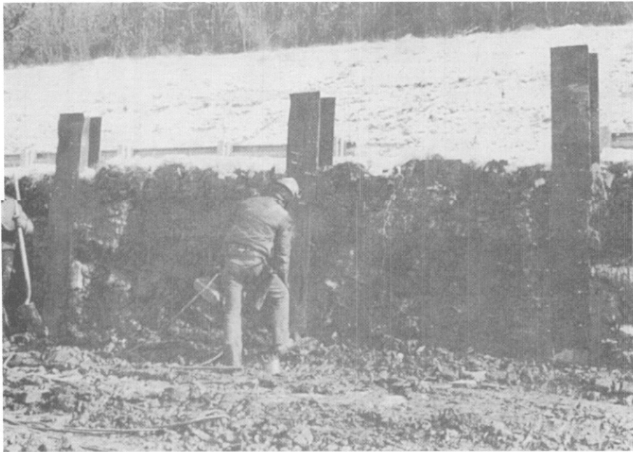
Figure 8. Piling in Place and Excavation of Embankment.
