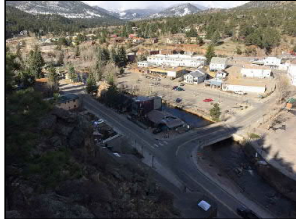
Big Thompson River and East Riverside Drive Corridor
