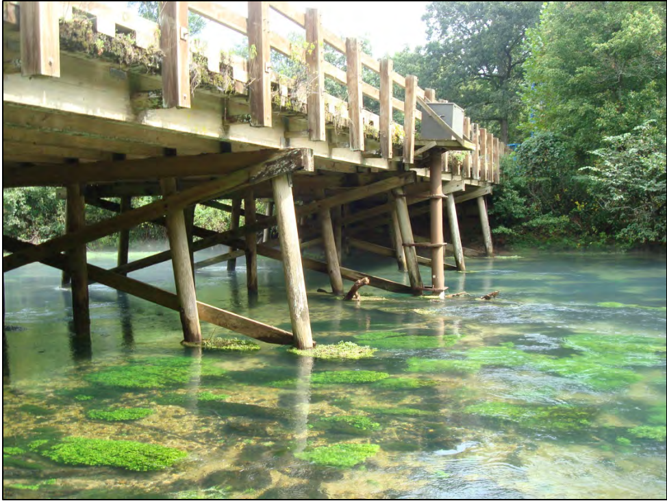
Figure 8. NE Corner of the Bridge
