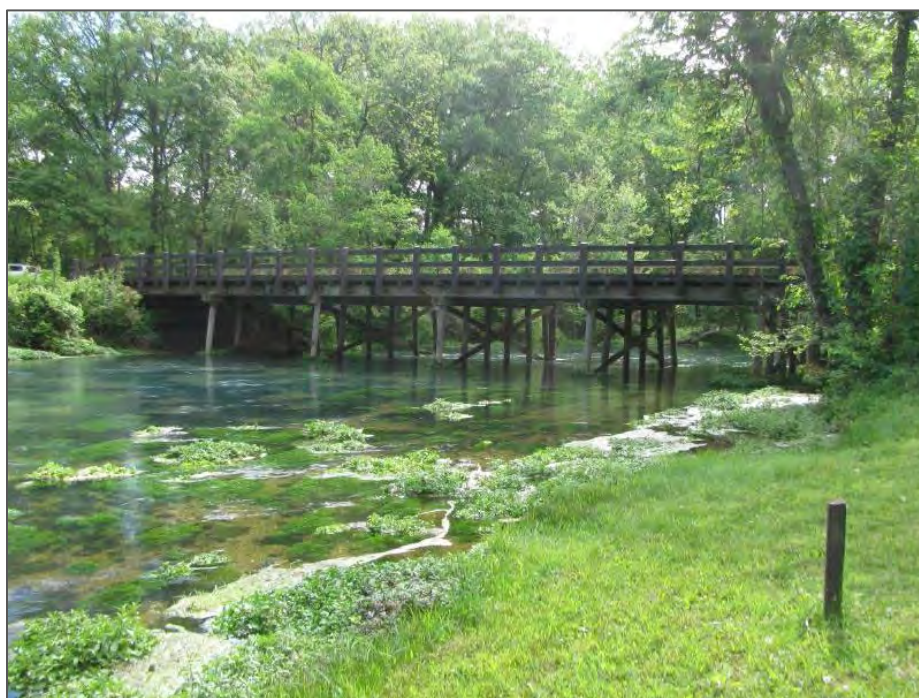
Figure 2. Existing timber glulam Big Spring Bridge
