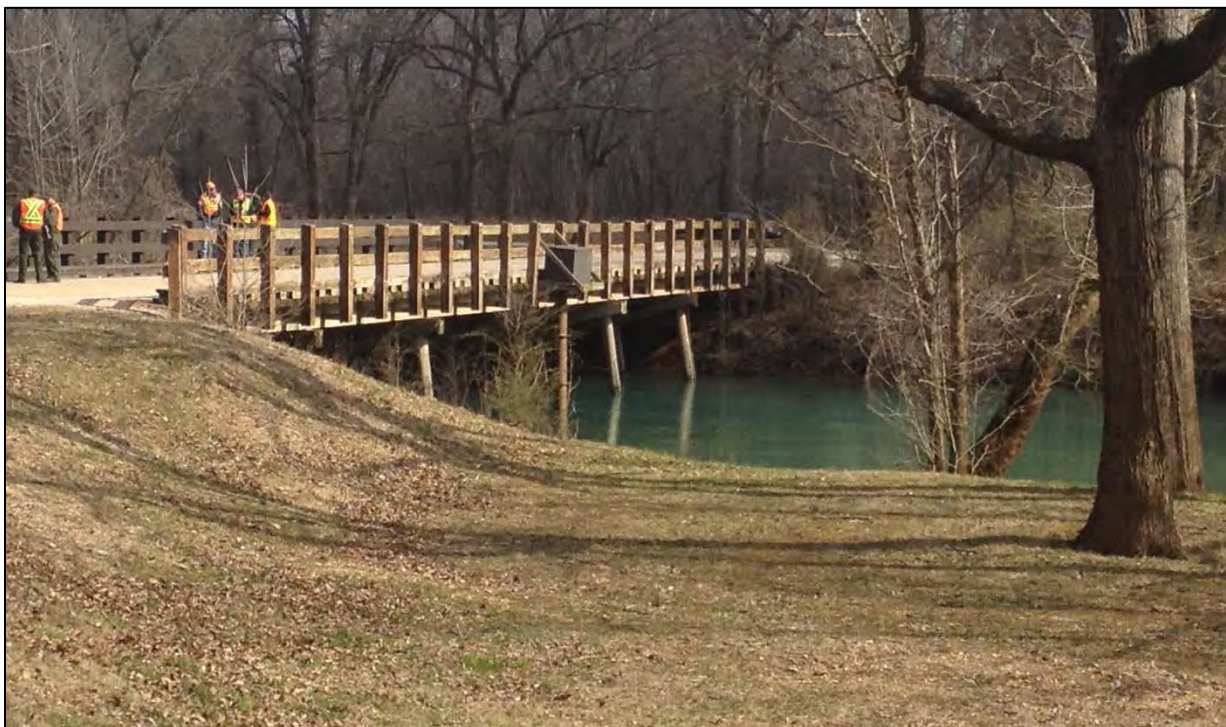
Figure 2. View of Big Spring Bridge Showing Bridge Approach In Relation to Surrounding Landscape
