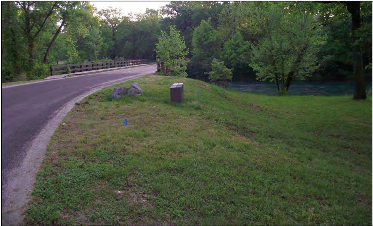
Figure 3. View of Opposite Bridge Approach
