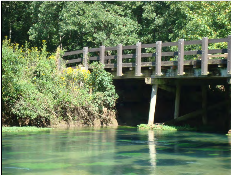
Figure 6. NE Corner of the Bridge
