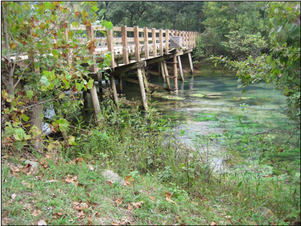
Figure 9. SE Corner of the Bridge
