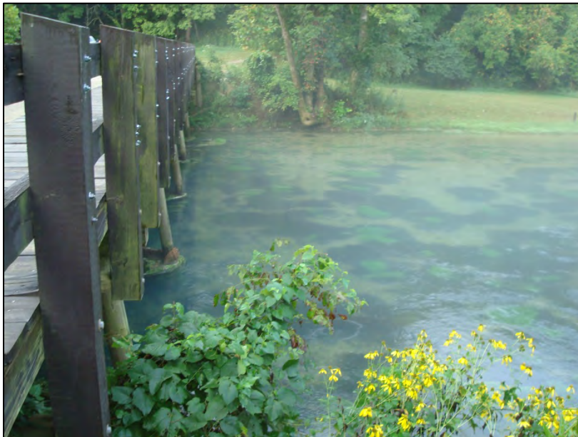
Figure 7. SW Corner of the Bridge
