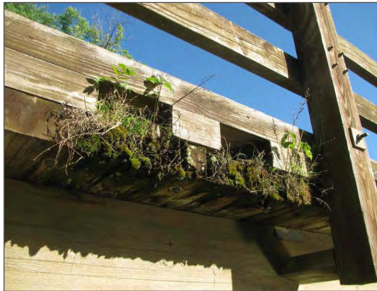
Figure 3. Typical decay of deck panel edges with vegetation growth present.
